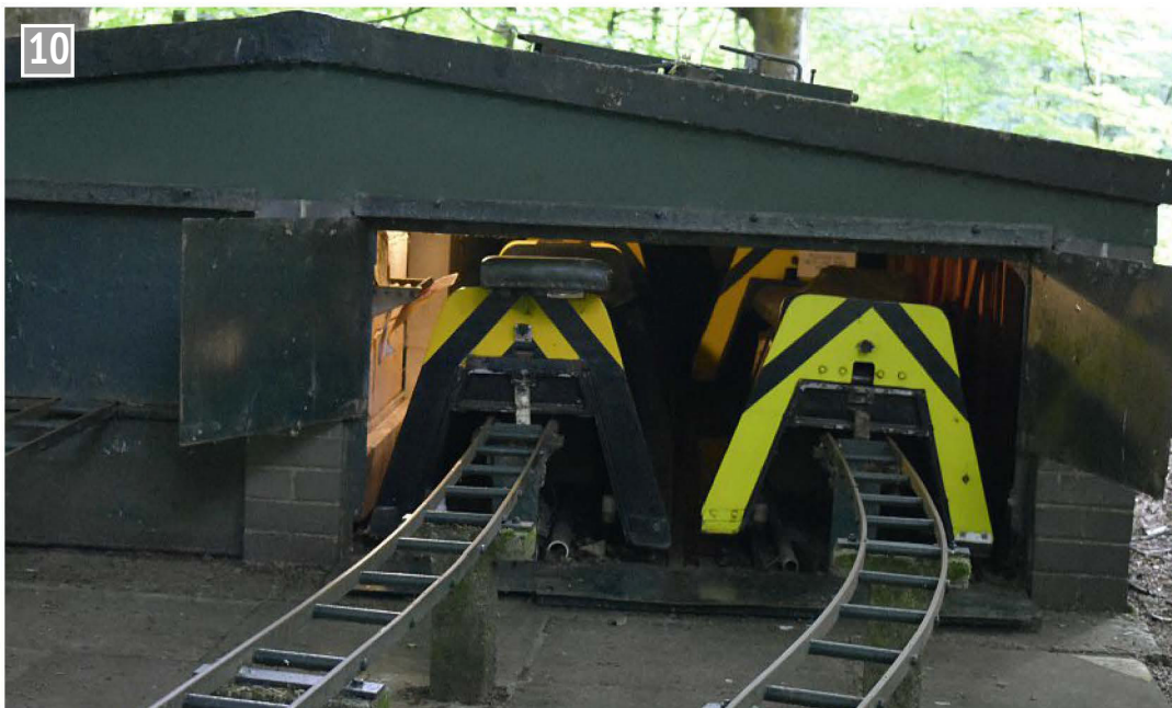
Inside the compact carriage storage shed.
