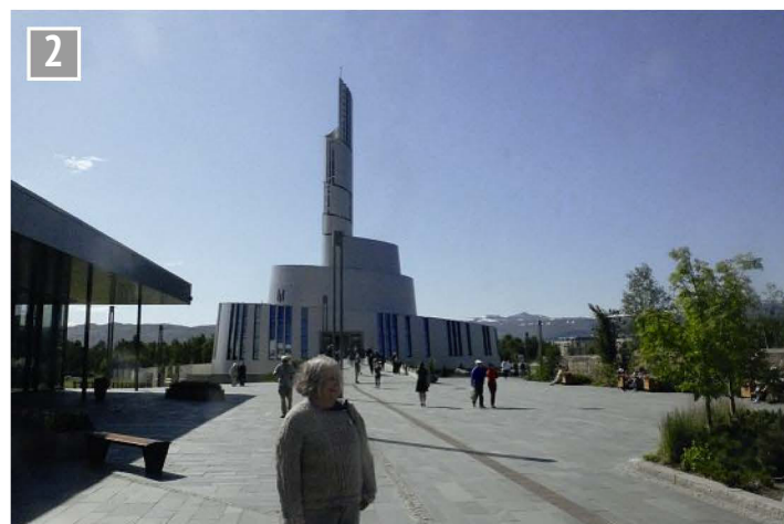
Northern Lights Cathedral, Alta.
