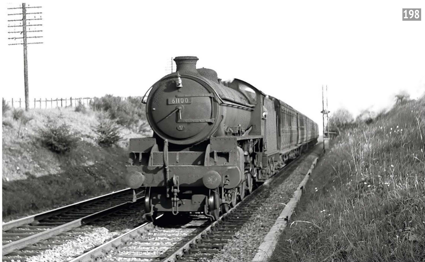
Early smoke box door on 61100 (photo by Rail Photoprints).
