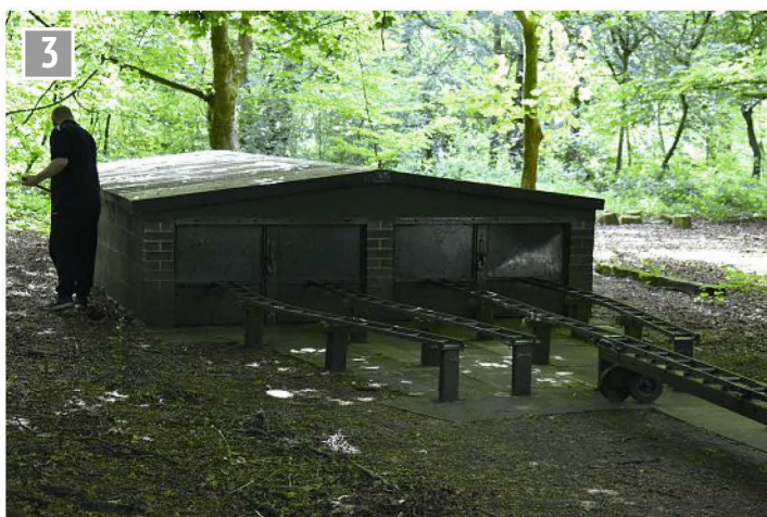
A low level stock shed receiving some attention.
