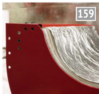
The cover plates lightly pinch the insulation and aluminium foil, holding everything in place.
