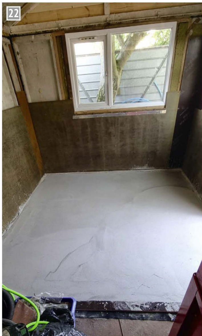
Levelling compound when cured.
