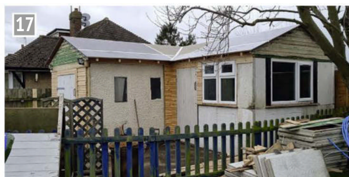
A start is made on the new roof, with plywood sheets.
