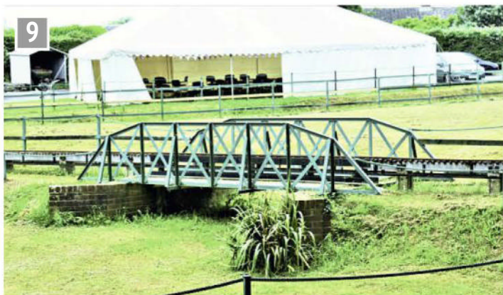
The excellent string girder bridge across the middle of the site.
