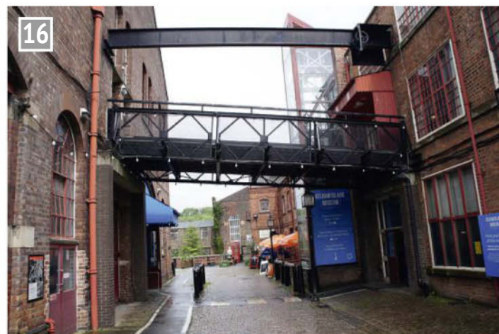
16 This example of a Bailey Bridge links two museum buildings. Such bridges were an essential part of the Allied advance in Italy during the Second World War.
