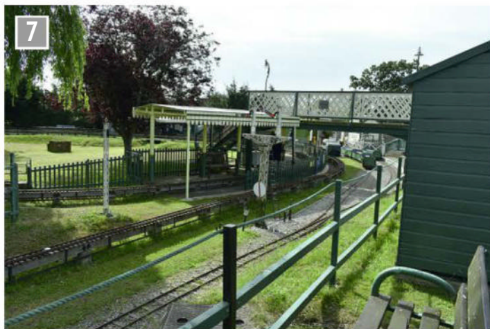
The station approach and footbridge.
