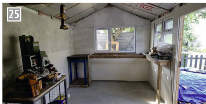
The first coats of paint are applied.
