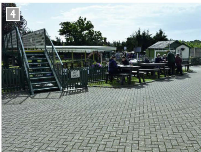
The paved area in front of the clubhouse and access to the footbridge.
