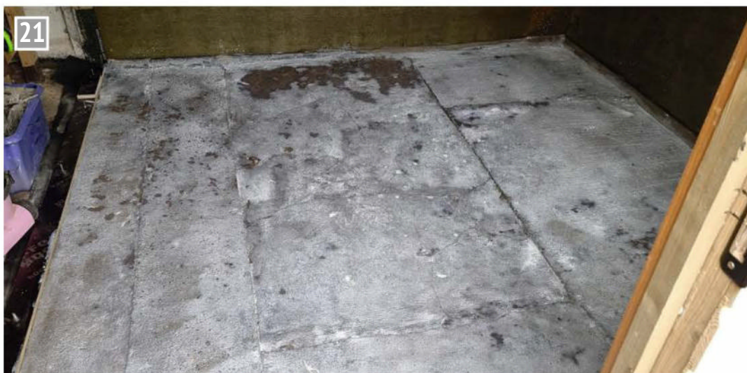
Partition board (left) separates the floor areas for levelling.
