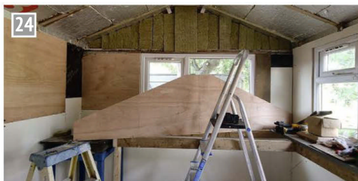
Fitting the gable end board.
