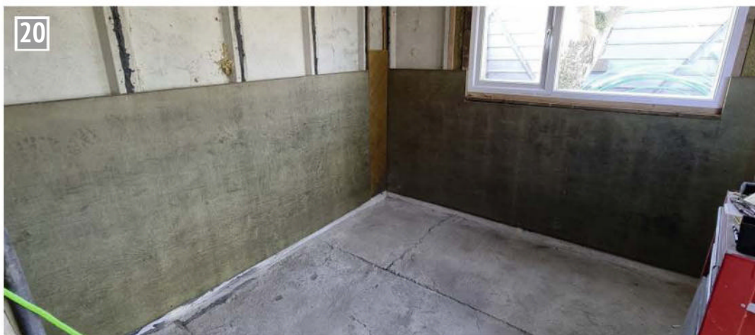
The lower part of the wall lining is done - time to level the floor.
