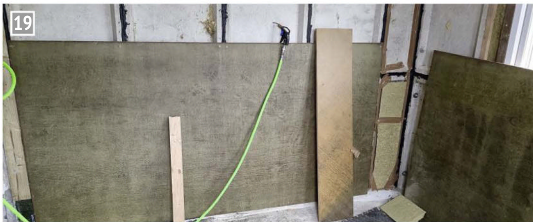
A start is made on lining the walls.
