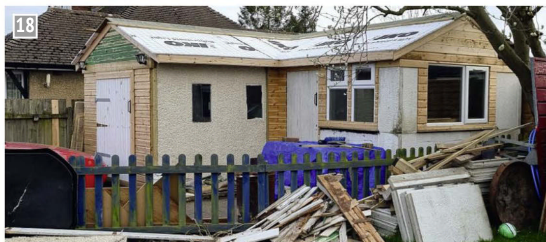
Waterproof membrane is added.
