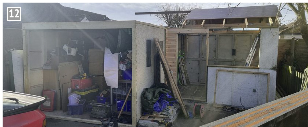
The extension to the garage is now well advanced.
