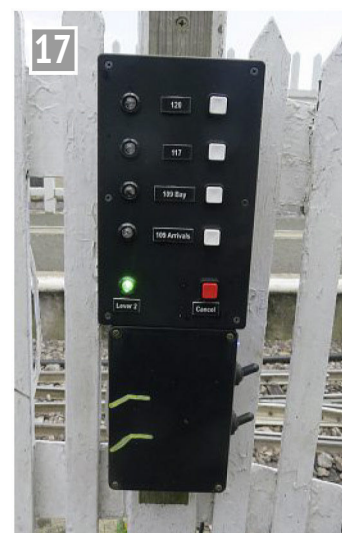
This pushbutton is Much Natter 109, 117 and 120 signals. The white buttons are 120, 117, 109 bay and 109 arrival.
