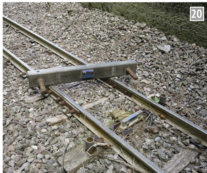
Barrier removed, to allow shunt out of siding.
