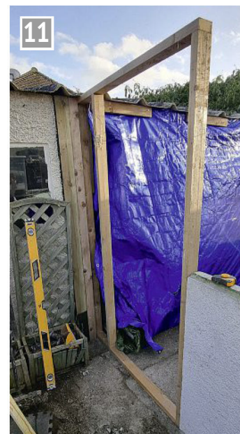
Frame dry fitted to check the fit.
