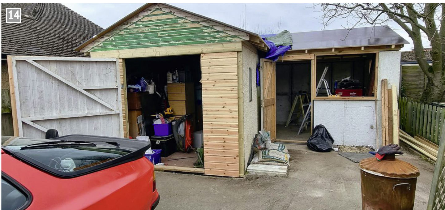
Further progress – doors fitted.
