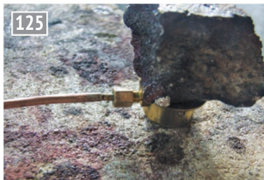
Here the pressure gauge is being protected whilst the pipe nipple is silver soldered to the feed pipe.
