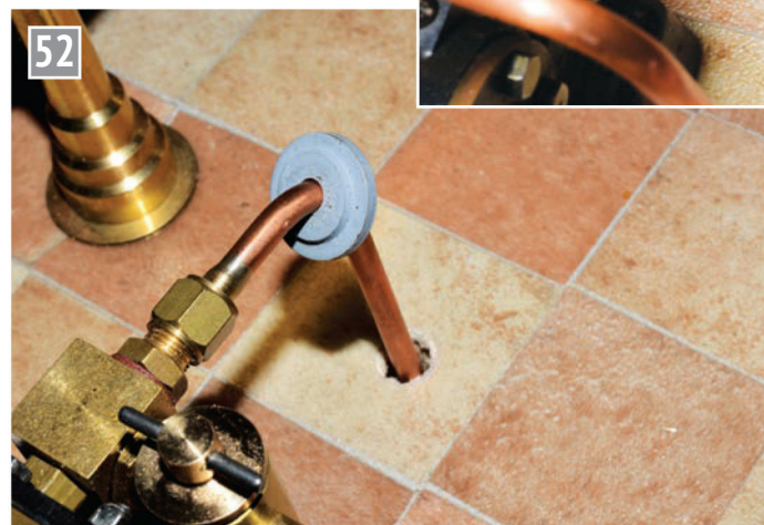
Covering a large hole in the baseboard with a washer.
