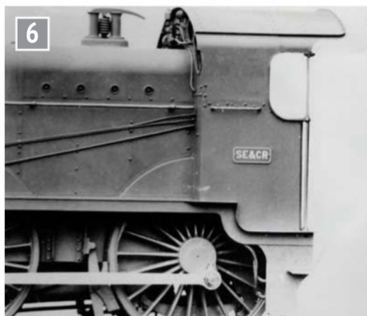
A D1 class in unlined grey livery with the SECR owner's plate as fitted during WW1. The D1s were Maunsell rebuilds of the earlier Wainwright D class.
