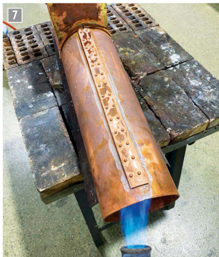
The boiler butt strap ready for soldering.
