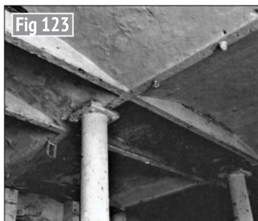
Fig 123 Parallel cast iron beams in iron framed building. The hatch between floors lies between the columns but was boarded over at the time that the photograph was taken. Lifting eyes and bolts set into main transverse beams. Survey by Structural Perspectives in 2005.
