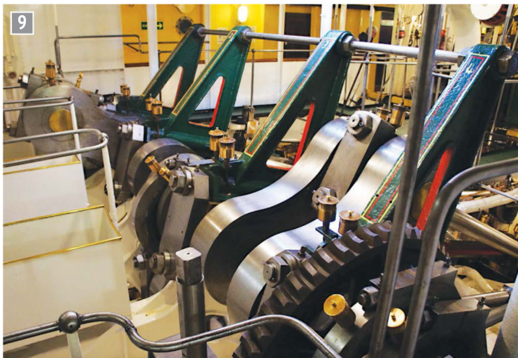
The worm wheel in the foreground is used to turn the engine over during winter to prevent pistons seizing in the cylinders.
