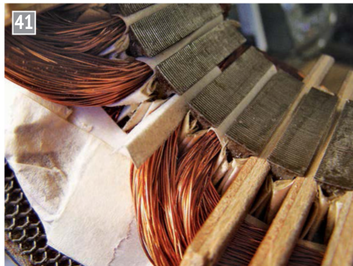
Fitting a slot closer with the inter-phase insulation fitted and held in place with masking tape.
