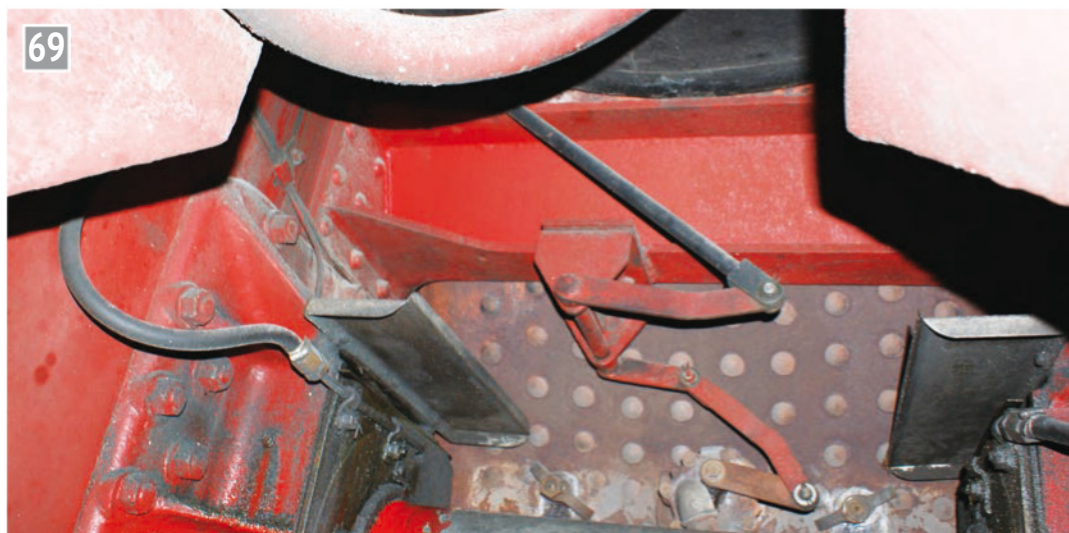
69 Blowdown valve and operating linkage.
