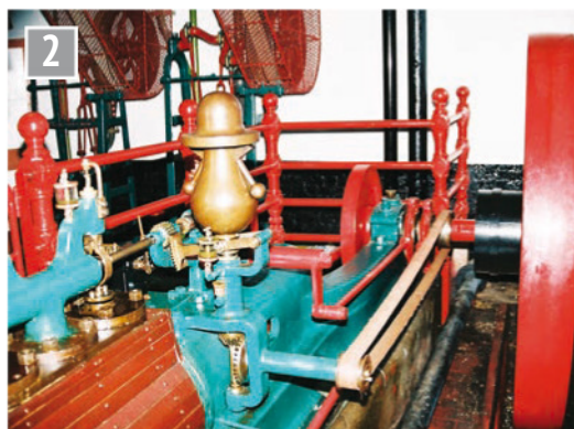
Hook Norton brewery - the last commercially working steam engine (now steamed occasionally) made by Buxton and Thornley.
