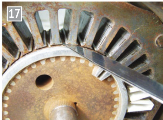
Measuring the air-gap using feeler gauges.
