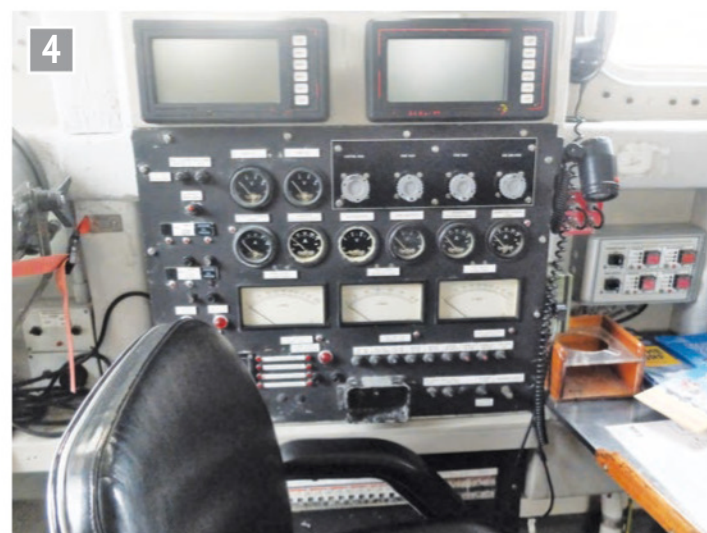
Engineers' panel, RNLI Lifeboat in 'Sheffield Bah't Shore'.
