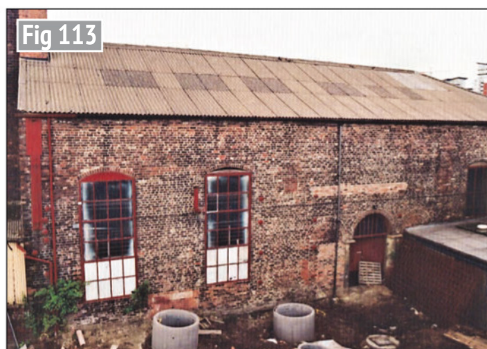
Fig 113 The East Elevation of the Drysand Foundry immediately prior to restoration in 2005. Survey by Structural Perspectives in 2005.
