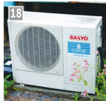
An air source heat pump is a comparatively efficient way of heating buildings. York Model Engineers installed one to heat their new workshop and are pleased with its performance.
