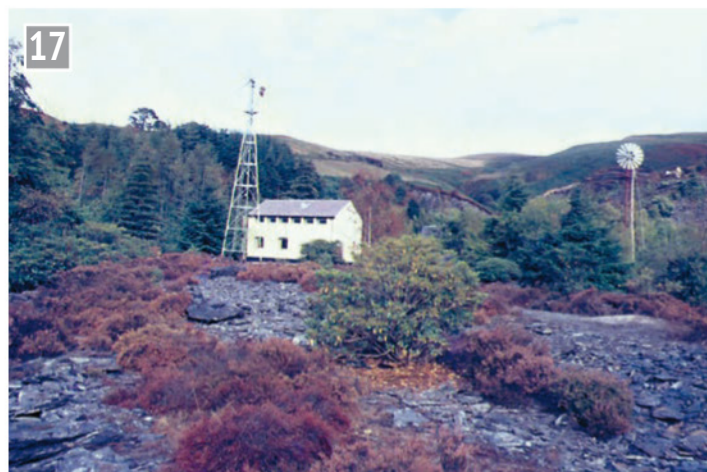
As it was.... The Wates House was claimed as the best insulated house in Britain when it arrived at CAT in 1975. (Courtesy CAT 2022.)
