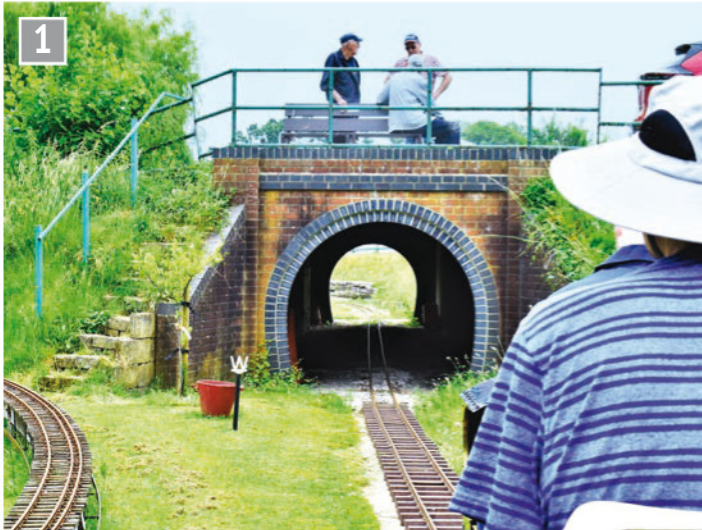
Drivers eye view of the approach to the tunnel on the ground level track.
