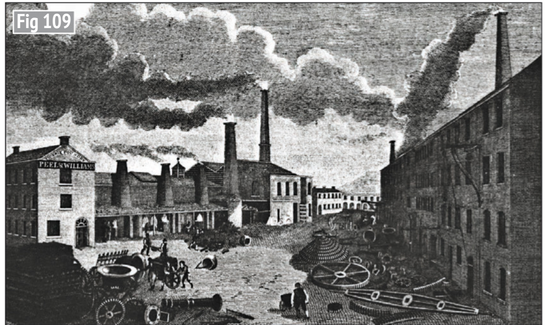
Peel Williams' Phoenix Foundry in Ancoats, Manchester. The left-hand building is the foundry with its open front and its furnaces.
