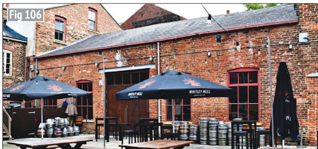
Murray and Wood's Greensand Foundry following restoration (photographed by the author in 2021).
