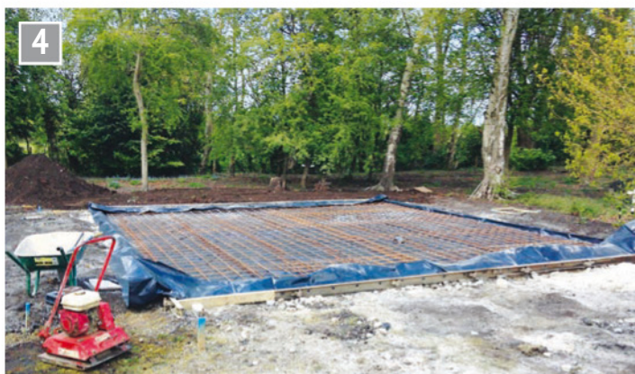
4 Concrete floors were the only parts constructed by external contractors (photo: Paul Howard).
