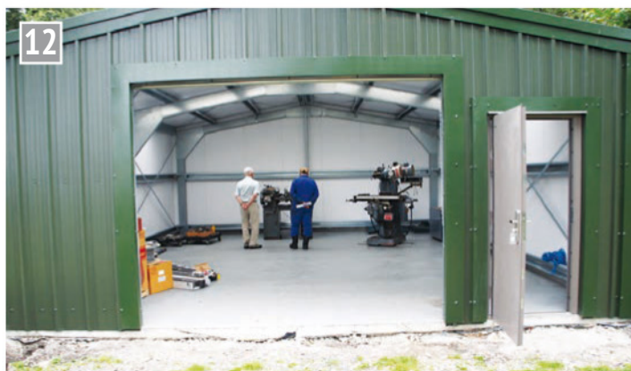
12 Fitting out started soon after completion, the workshop is spacious compared to the old shed.
