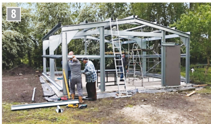
8 Pillars and roof girders assembled for the workshop (photo: Paul Howard).
