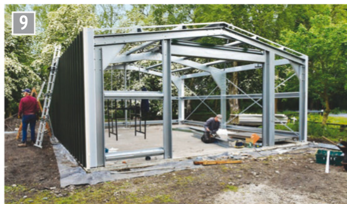
9 Side panels in place, building starting to look like a workshop (photo: Paul Howard).
