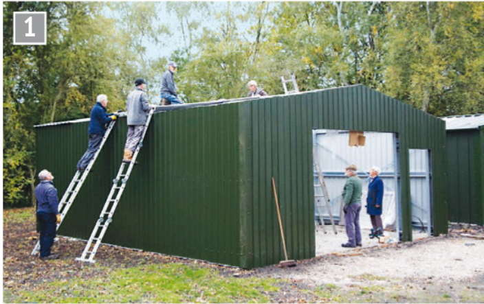
Two sheds built by York Model Engineers - workshop to the right, roof works ongoing to the new store on the left (photo: Paul Howard).
