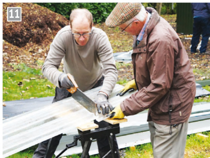
11 Although parts came ready to fix, some cutting to size was still required. Members trimming translucent roof panels to size (photo: Paul Howard).
