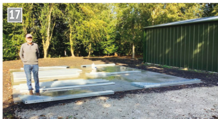
No let up here... Ted Burdge stands on the base of the new equipment store. Work started soon after completion of the workshop (photo: Paul Howard).
