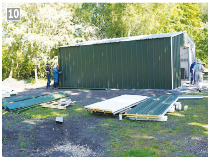
10 Fitting insulated side panels - the workshop can be surprisingly warm (photo: Paul Howard).
