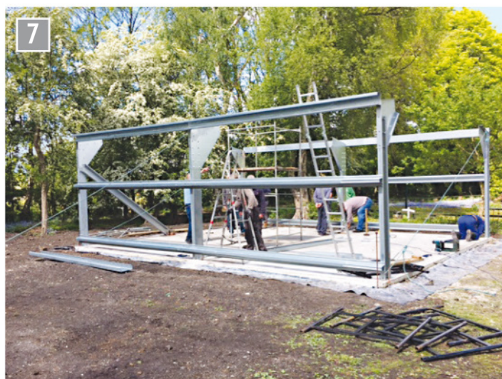
7 Workshop side frames erected; now for the roof girders (photo: Paul Howard).
