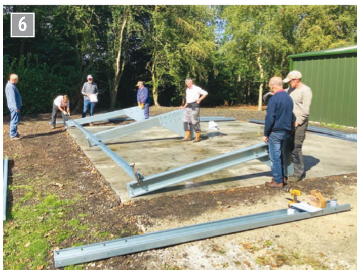
6 The erecting team get ready to put up one side of the new store. As with the workshop this was 'like assembling giant Meccano' (photo: Paul Howard).
