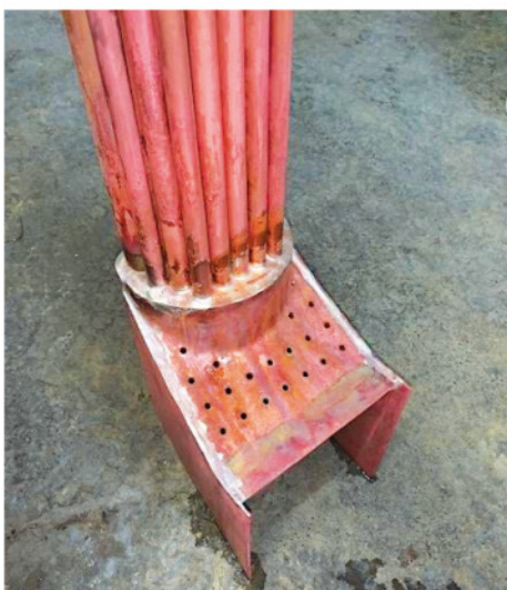
4. Here are the combustion chamber tubes. Larger pipes have been installed for a better tube/grate ratio.
