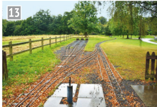
The arrival side of the ground level track showing the three sidings and moving sector plate.
