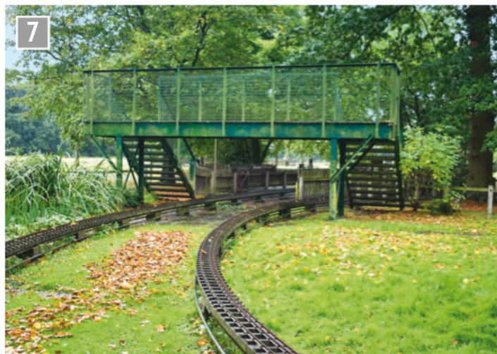
The substantial footbridge over the raised track.
