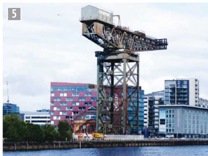
Well known Glasgow landmark, the Stobcross or Finnieston crane was used for loading cargo including locomotives from Springburn. Built by Cowans, Sheldon of Carlisle and Cleveland Bridge of Darlington it is 53m high (175 feet) and could hoist 175 tons. Unusually it has an auxiliary hoist for lighter loads. An entrance to a former Clyde tunnel is just behind the crane.
