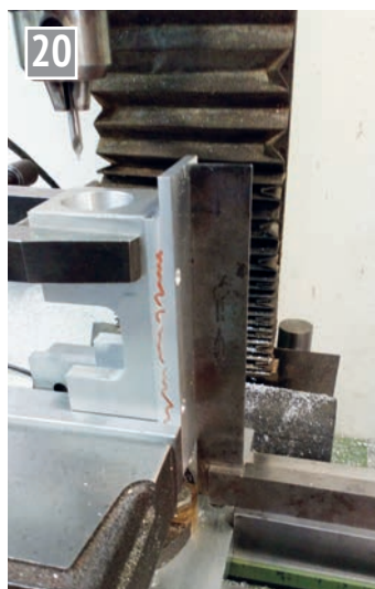
Drilling the holes for fixing the front to the sides.
