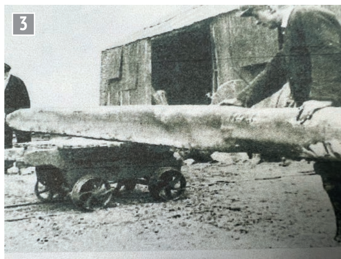
Crushed pipe from the oil well.
