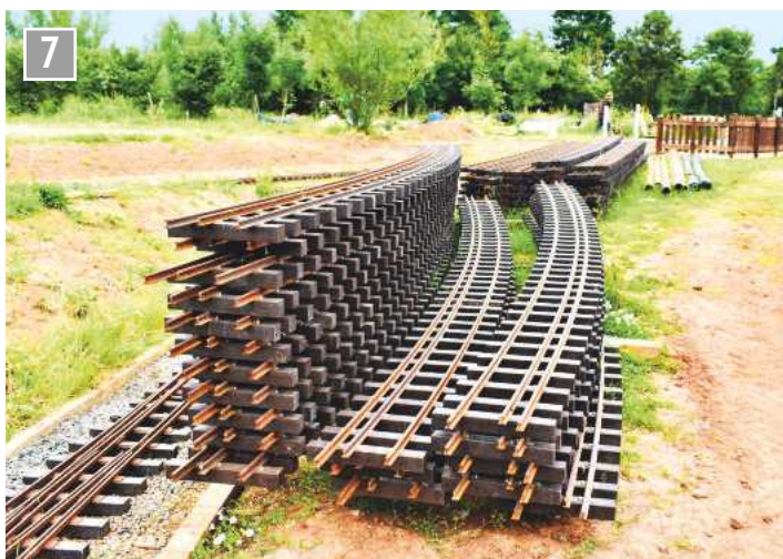
Track panels ready for laying.
