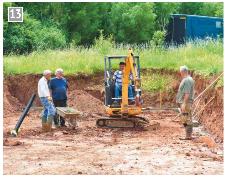
Work on the carriage shed continues.
