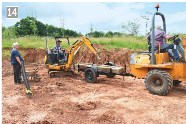
Concrete sleepers being unloaded for the footings.
