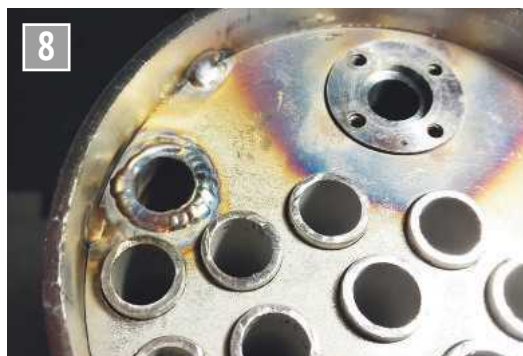
Welding the tubes to the smokebox tubeplate.
