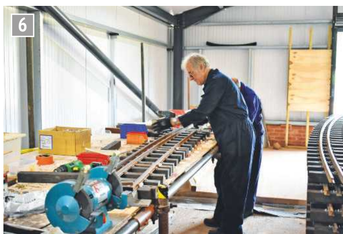
Members busy constructing track panels.
