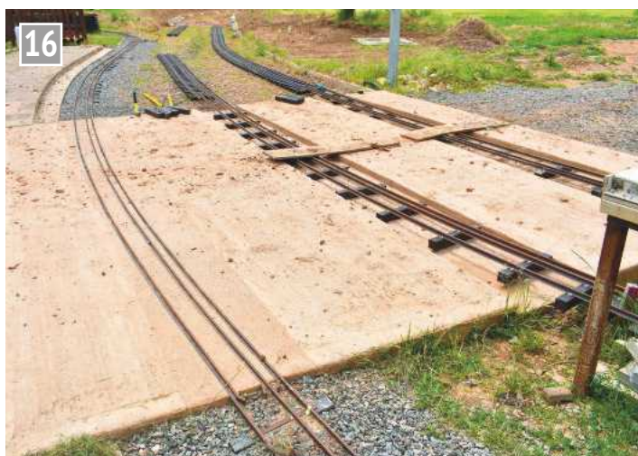
The road crossing in place but awaiting the finishing touches and gates.
