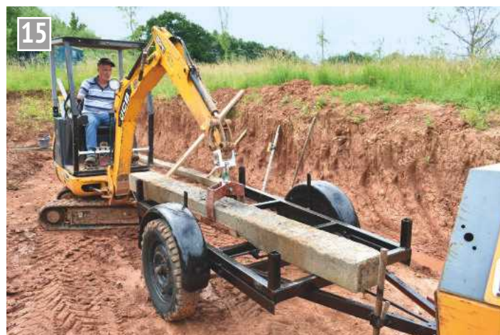
Chairman, David Hartland grabs the next sleeper for the footings.
