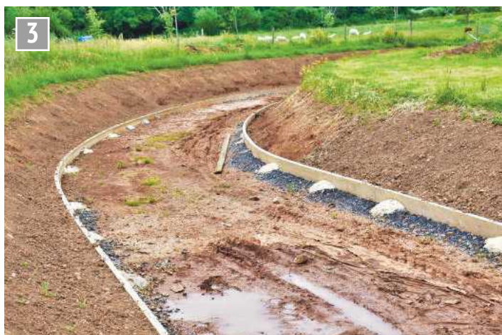
View showing the superb ground works for the new track, neatly battened embankments and edging boards.
