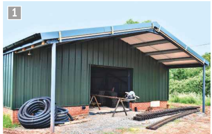
The south-east end of the new building showing some ground water pipework and yet more track panels.
