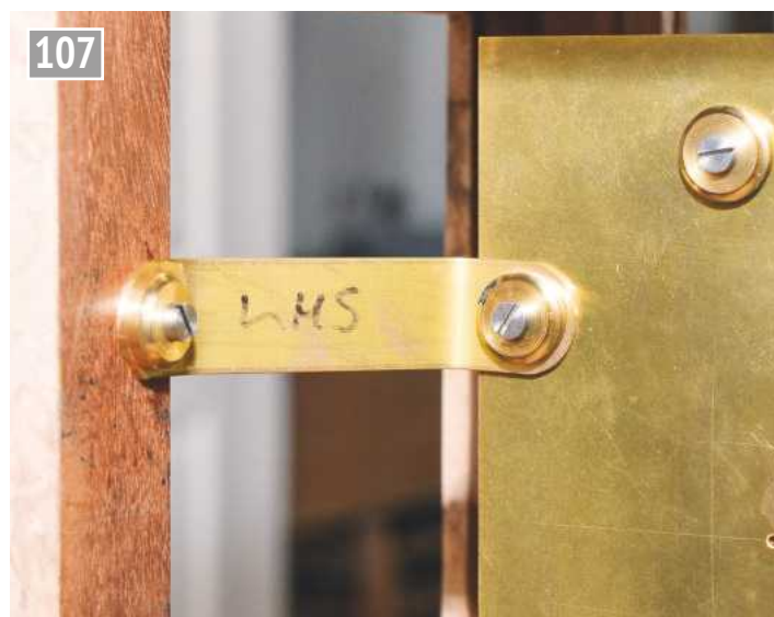
Fixing the upper brackets.
