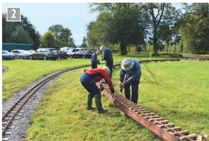
Husband and wife team, Steve and Alex Bouchard working on the track fixing sleepers.
