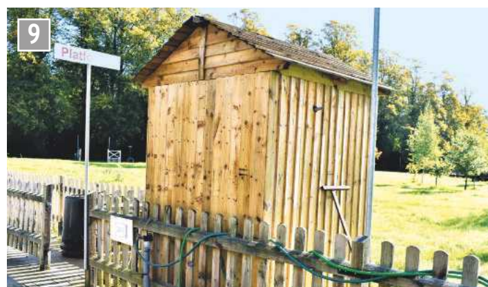
The main water pumping shed on platform 1.
