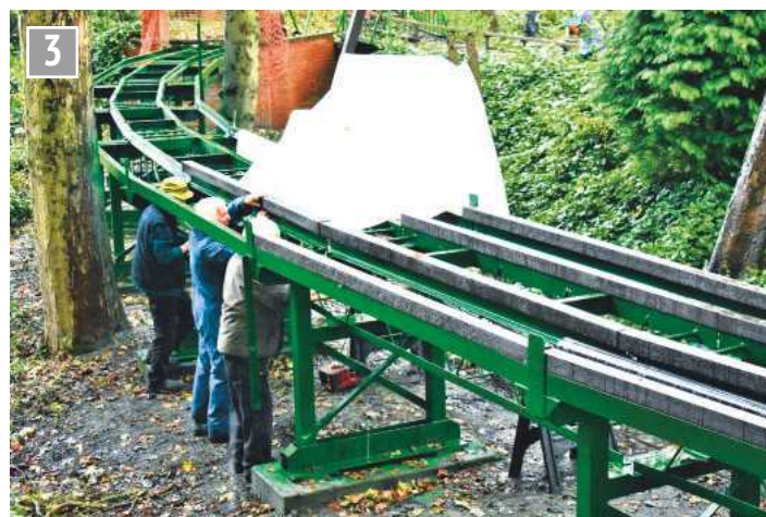
Members working on replacing timbers on the refurbished viaduct.
