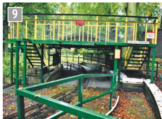
The substantial footbridge over the raised track station area.
