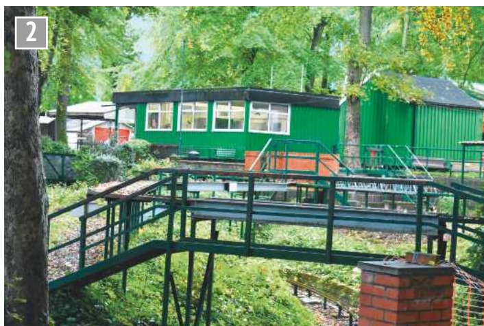
The footbridge over the raised track adjacent to the viaduct.
