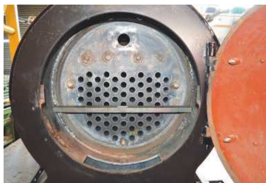
Blyth's smokebox tubeplate is seen in this view. The steam pipe header has yet to be fitted.
