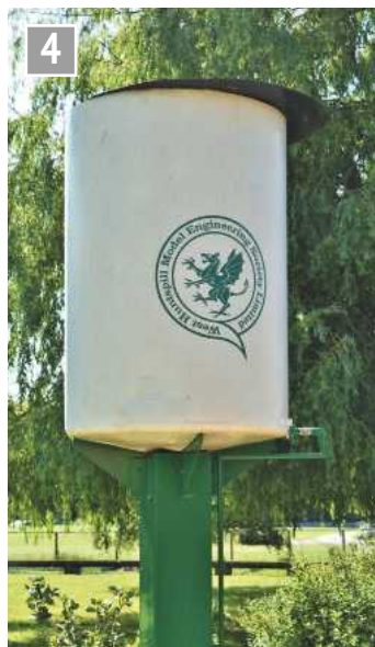
A good size water tower serves the station area.
