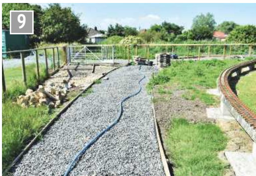
The prepared track bed approaching the proposed road crossing.
