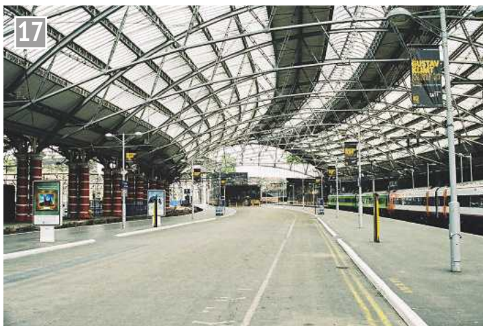
17 Lime Street Station is a fine gateway to the city with a magnificent sickle truss roof.
