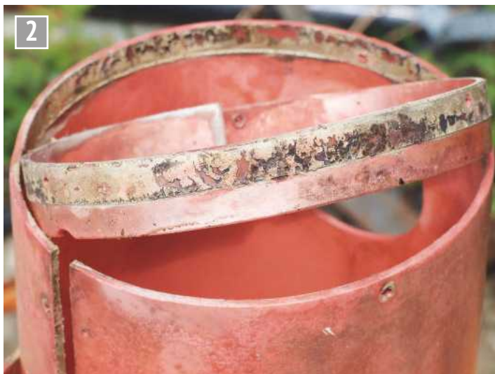
Oh dear – evidence of poor penetration on this ring.
