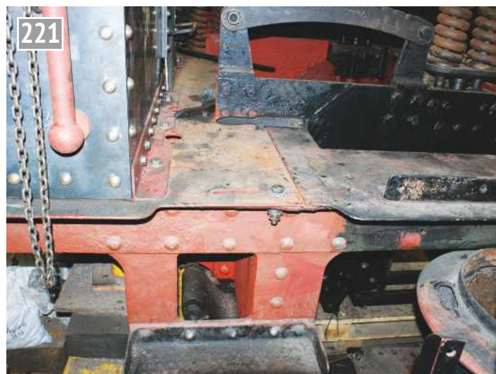
Joint in the platform, extending across the cab.
