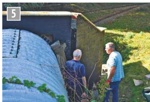
Members putting the finishing touches to the back of the tunnel portal before it is covered in soil.
