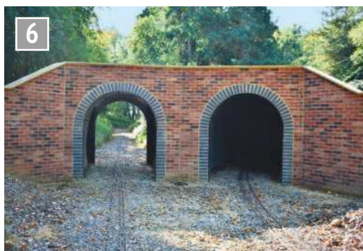
The double tunnel portal on the one short and one long tunnel.
