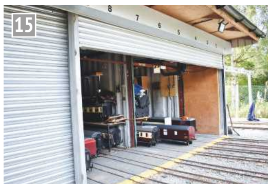
The standard gauge carriage storage shed.
