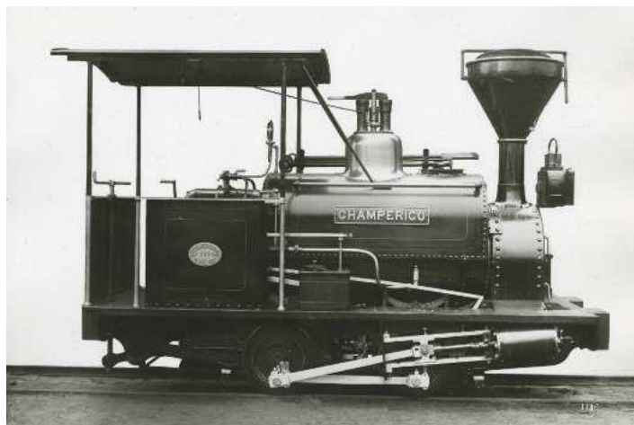
Inside framed variants of the dynasty intended for wider gauges than nominal 2ft continued to be constructed after Little Egret and this 3ft gauge variant, Chamerico, apparently incorporating Peep-o'-Day (or similar) - pattern boiler, cylinders and motion was dispatched on December 14th 1883.
