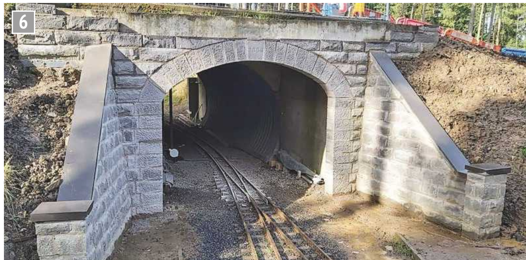
The road bridge at Almondell (photo courtesy of Robert McLuckie).
