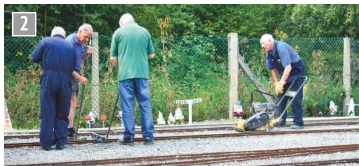
Track maintenance gang at work on Old Oak yard.
