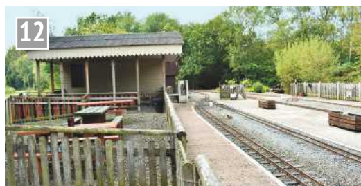
The four road Far Leys station and water tower.
