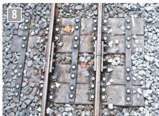
The secure and complex track circuitry locations.
