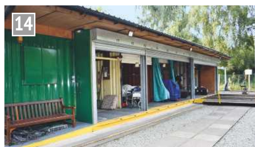
The full set of storage buildings.
