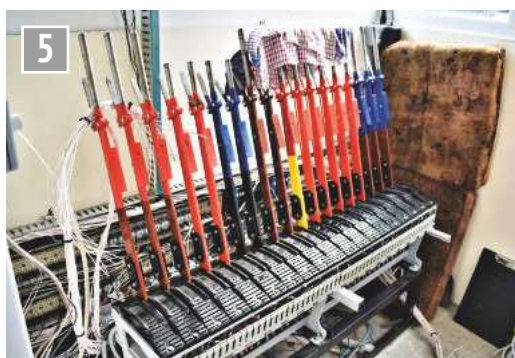
Awaiting completion of the circuits in Harvesters Middle Box.
