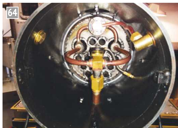
Inside the smokebox.
