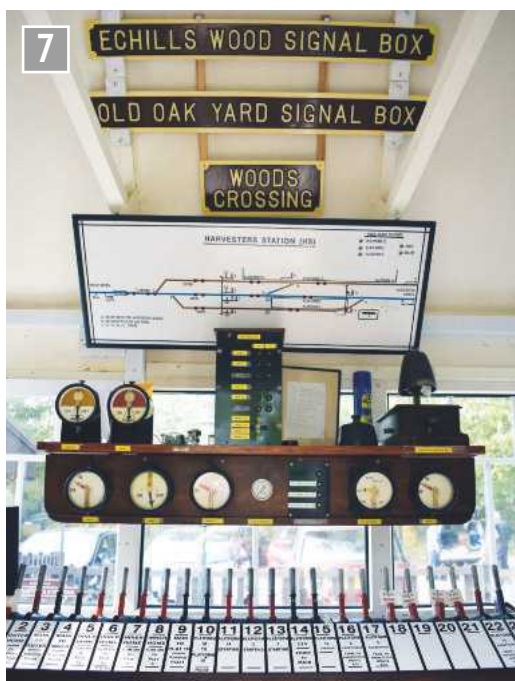
Lever frame and track diagram in Station Box.
