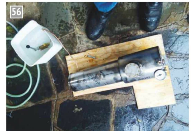
Boiler pressure test.
