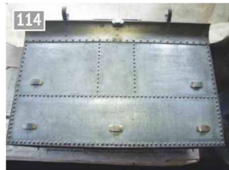
114 All the rivets have been carefully peened down here and in some cases a small punch was needed to get them flush.
