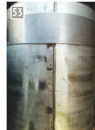
Clamping the barrel for welding.
