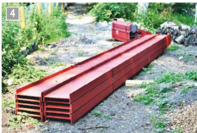
New steel sections for the bridge deck.
