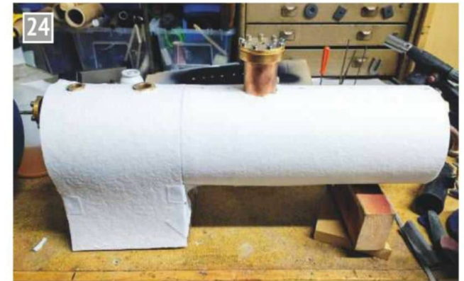
Glass fibre insulation in place.
