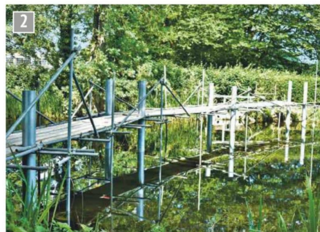
Scaffolding and supports for the new bridge await the installation of the steelwork.
