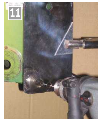
Using the mirror to guide the drill.
