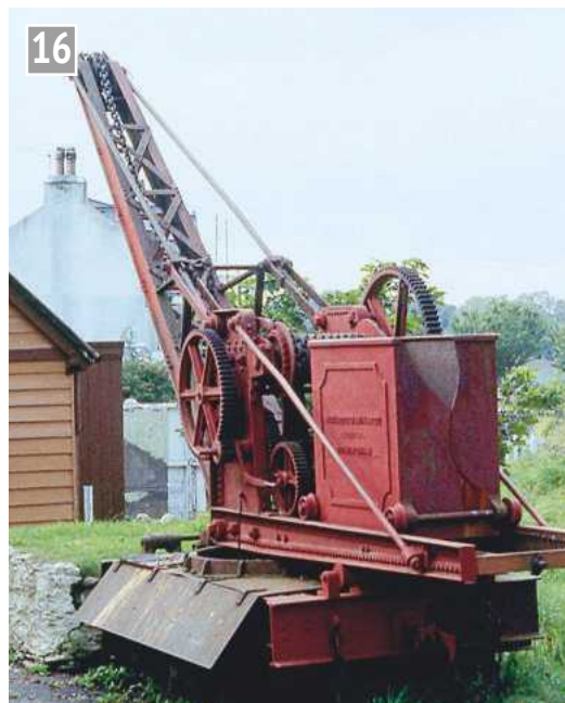
Travelling crane seen in 1980. Built by Richard C. Gibbins and Co. in 1893, now preserved at former Union Mills station. (Photo: Roger Backhouse 1980.)
