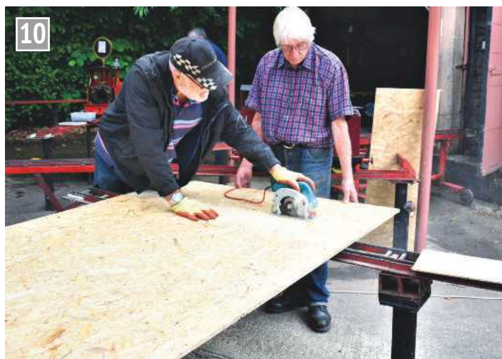
Preparing the next panel for the new storage shed.
