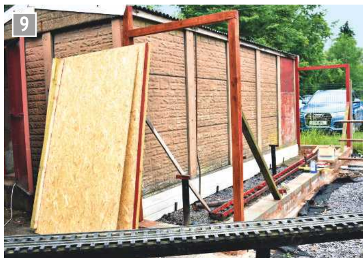
The new shed under construction.
