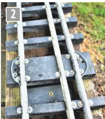
LEFT: A section of track fitted with the new plastic sleepers and the track circuit connections in place. RIGHT: The sleeper gang milling machine has six spindles.
