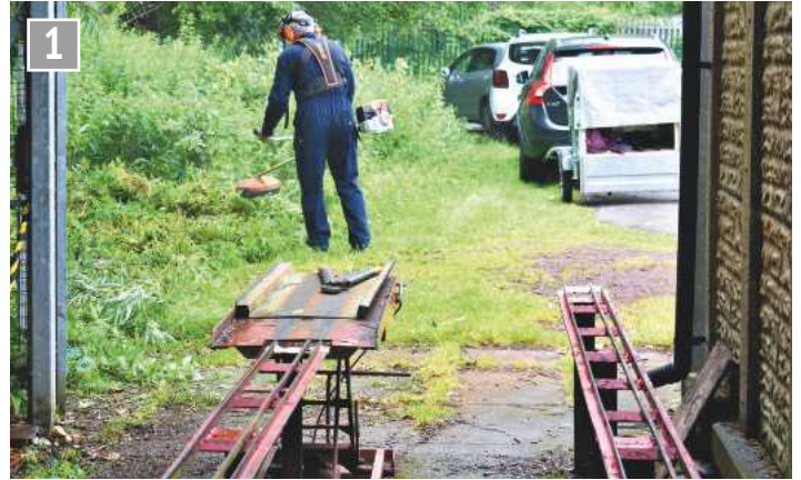
Clearing weeds and undergrowth outside the loading bay.
