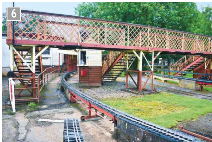
The fine footbridge giving access to the central picnic area.
