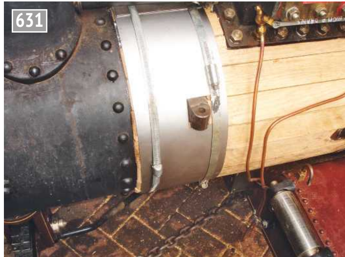
First sections in place.
