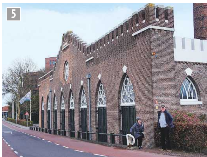
The former boiler house first housed Cornish and then Lancashire boilers. It's adjacent to the Ringvaart to ease the unloading of coal. This now houses the museum.
