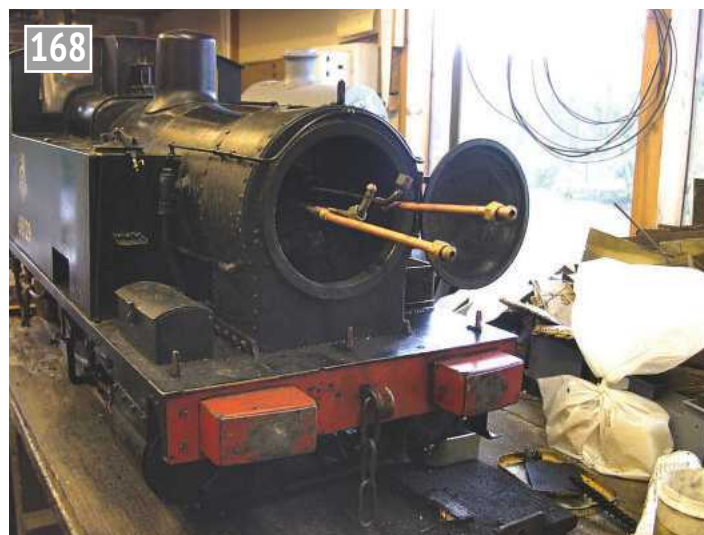
Installation of superheaters in the Y4.
