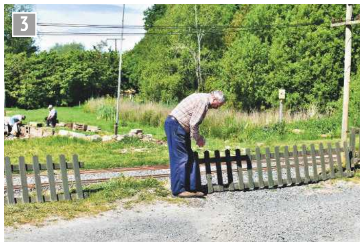
Chairman Wally Sykes repairing one of the flood damaged fence panels.
