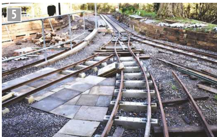
View from the tram shed onto the main line.
