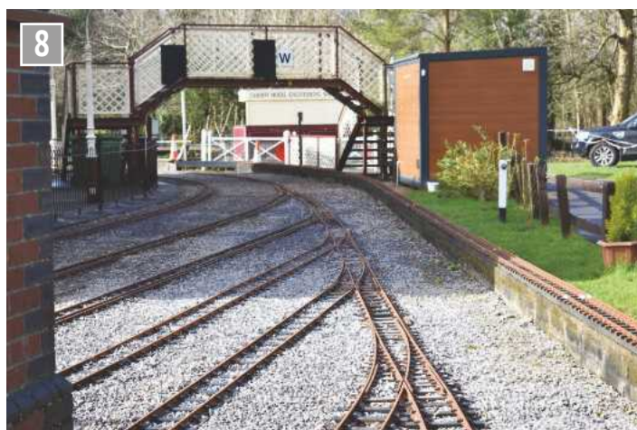
Immaculate trackwork through the station area.
