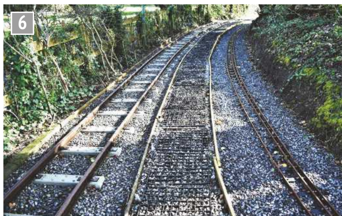
Side by side the new tramway and new dual gauge main line. The centre pathway has to be completed.
