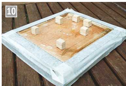
Preparing to cast a concrete base.
