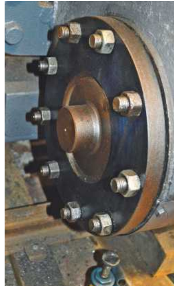
The leading left-hand cylinder cover required replacement. A repair in India had seen a piece of steel plate used in this role. The new cover, cast at a local foundry and machined on site, is seen in this view.
