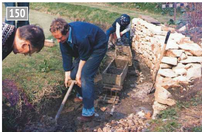
Digging out the cutting at Ais Gill.
