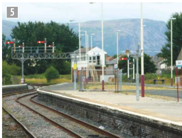
Llandudno signal gantry in July 2019.
