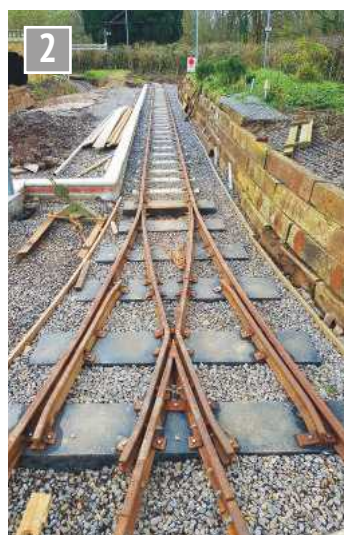
The tram line benefits from new concrete sleepers.
