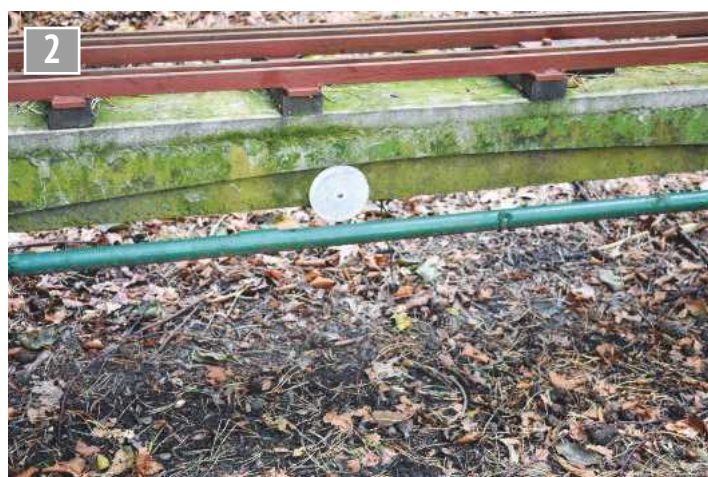
This shows the new surface skim to the old beams and one of the signalling light reflectors.
