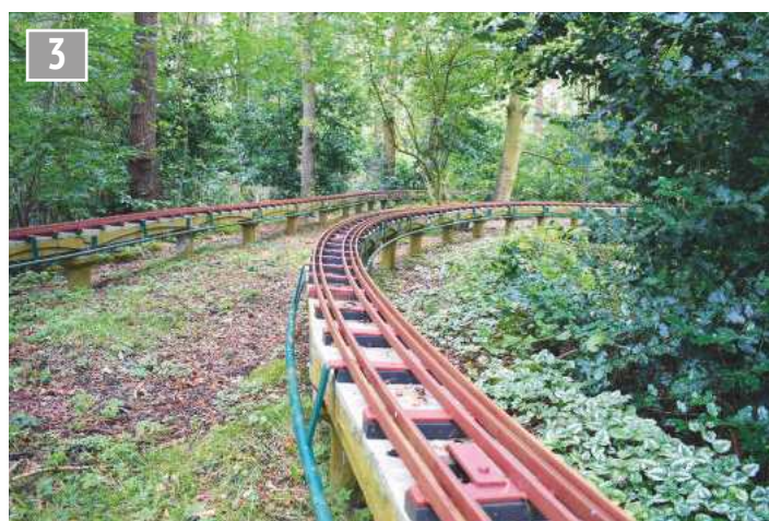
The super elevation built into the track base.
