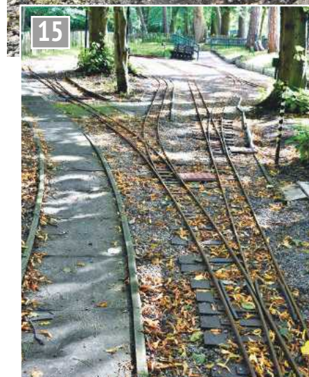
A four road low level station approach track work.
