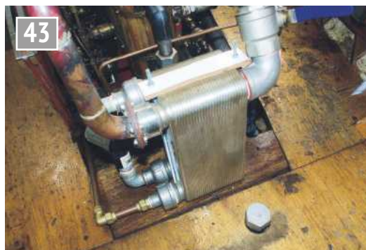
The inboard condenser.
