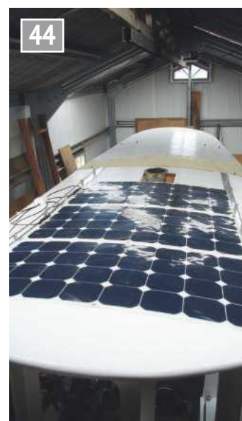
Flexible solar cells mounted flush on the cabin roof.
