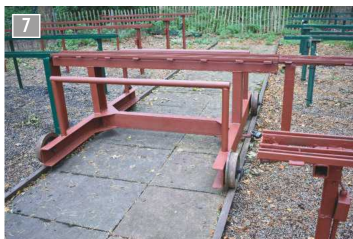
The substantial raised track traverser.
