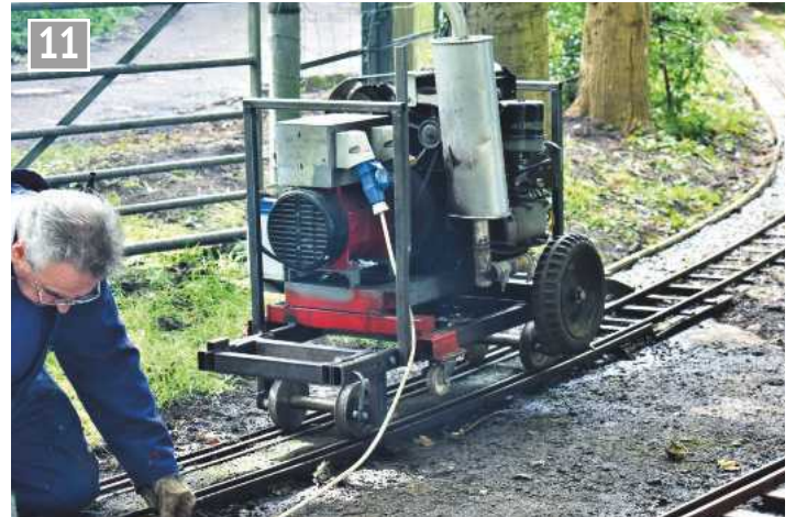
A well built high powered generator for welding at any location.
