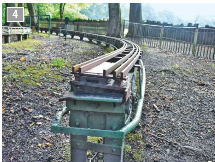
An end view of the new track showing the material section and anti-tipping rail position.
