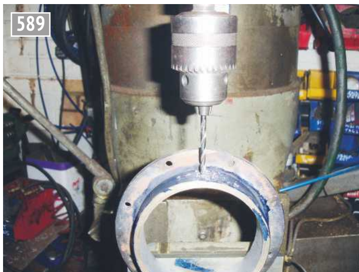
Drilling chimney base ring.
