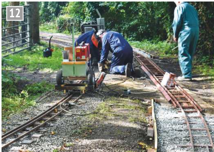
Members hard at work on the track crossing.
