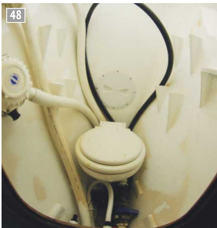
A marine toilet is shoehorned into the bows.
