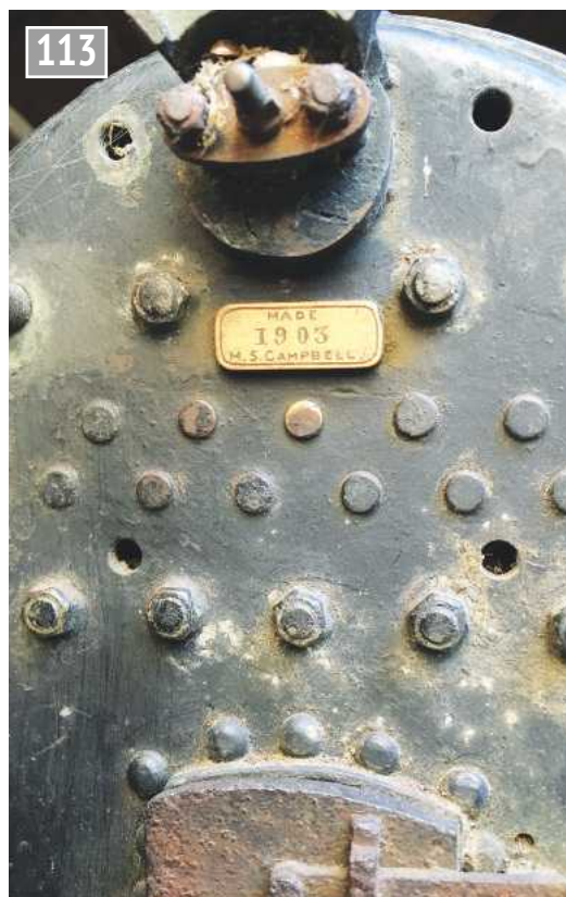
Original 1903 boiler backhead with maker's plate.
