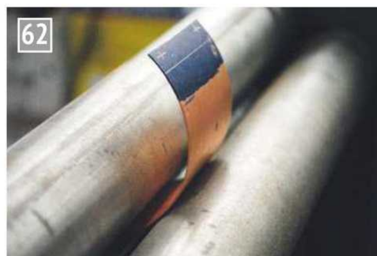
The cladding goes through the bending rolls.
