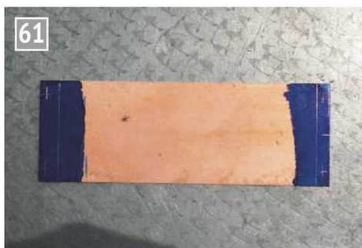
Cladding marked out ready for rolling.
