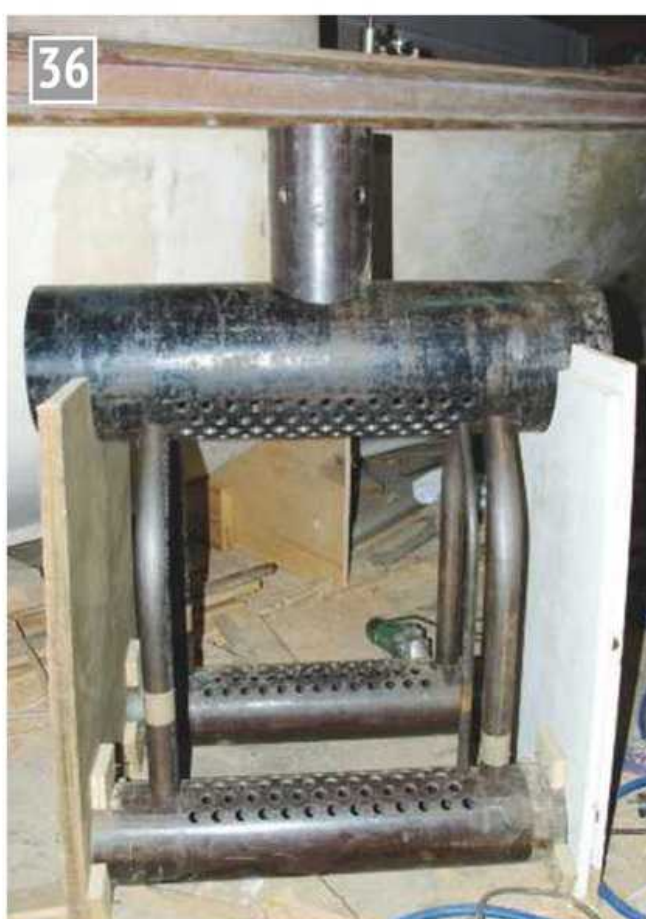
The tubes mounted in a wooden jig ready for welding.
