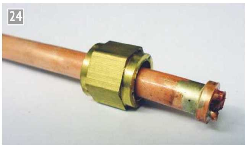
After pickling, ready for final cleaning up.
