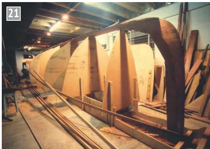
Formers and Keelson set up on hog ready for planking to begin.
