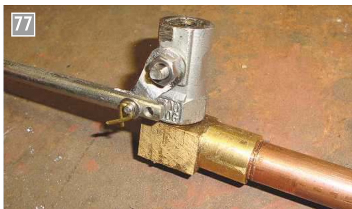
Regulator valve. A retaining pin was installed at the 'big end' after installation in the boiler.
