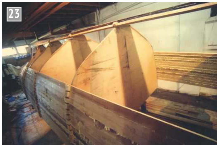
Planking in progress.
