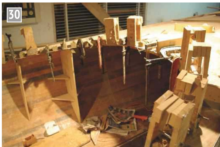
Laminating an edge around the coaming in situ.
