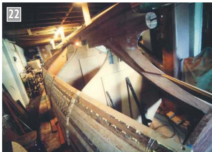
Planking has reached the round of the bilge. Note rebate on deadwood.
