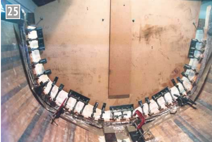
Laminating a rib in place.
