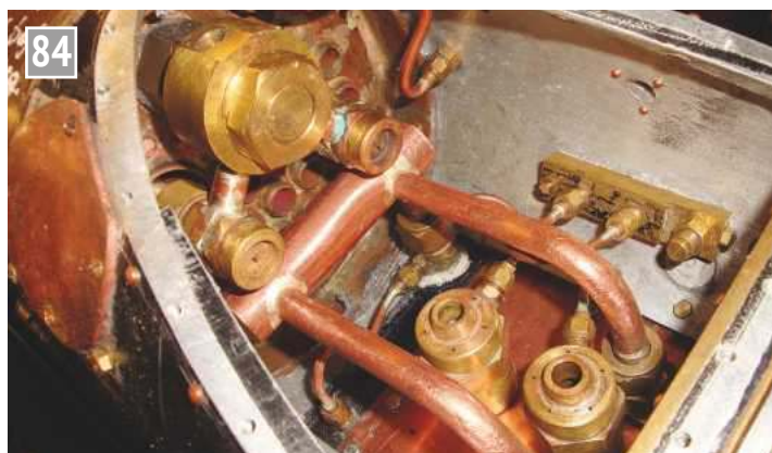
With the superheater installed, space is at a premium in the smokebox. The threaded hole in the top of the wet header is for the snifting valve. The hole in the side of the smokebox is for the vacuum ejector exhaust pipe.
