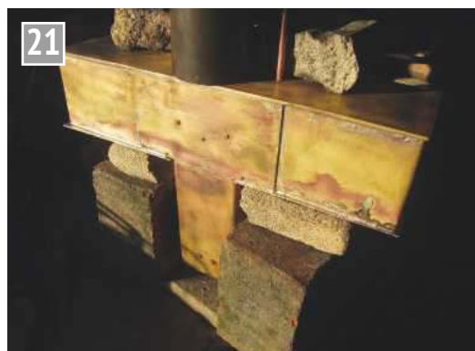
This shows the soldering task is reaching a conclusion and minimum distortion has occurred.
