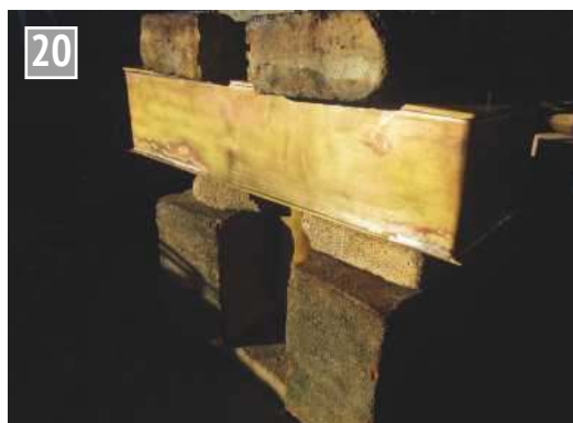
The tank is now turned over to solder along the edge of the bottom plate keeping the fireproof insulation just behind the edge of the sheet to allow the best heating condition.
