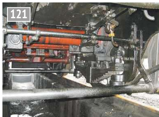
Another view of the drain cocks, looking backwards.
