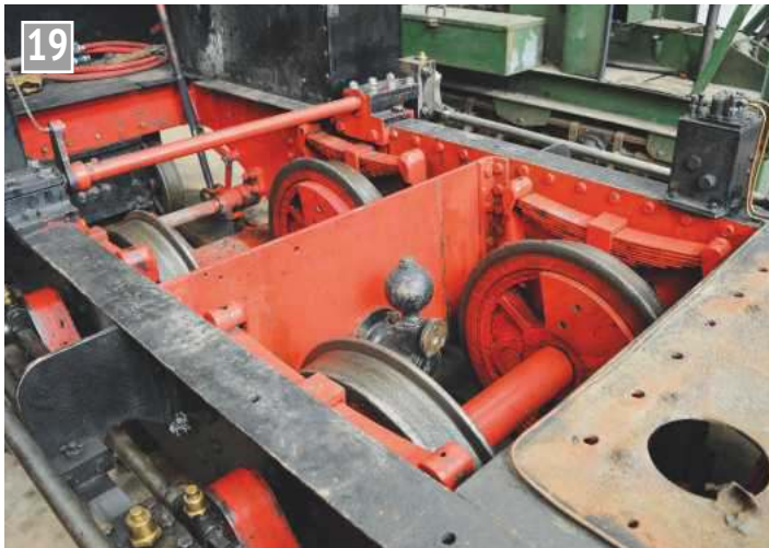
19 Stanhope's replacement coupled wheels came from a Hudswell Clarke Diesel locomotive and they are shown here in close-up. An original pattern feedpump has been fitted to the motion stretcher although this is not connected up as the engine now relies totally on injectors for water feed.
