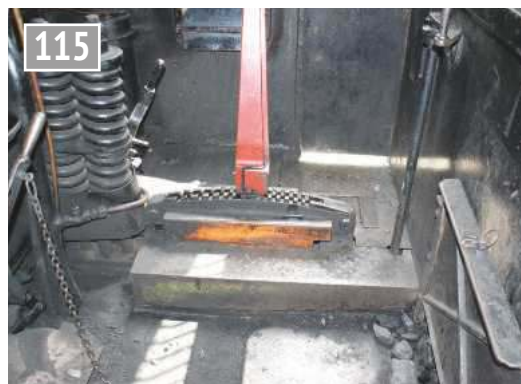
Drain cock lever (just peeping out from behind the springs).
