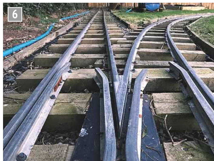
Philip Lockett's points at MES(NI) (photo courtesy of Philip Lockett).
