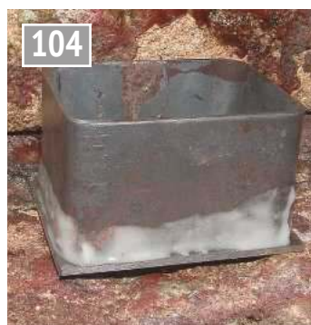
Soldering the bottom of the tank.
