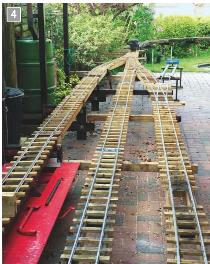
The reconfigured siding and a new head shunt on the loop.
