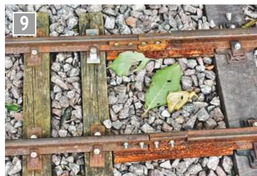
The simple but effective track transition section connecting the different weights of track.
