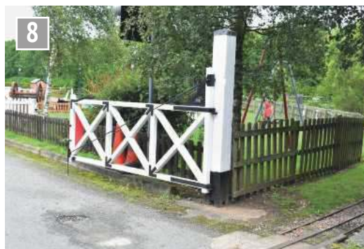
A new crossing gate on the extension, note the heavy duty road section.
