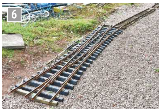
An impressive double slip installed at Parkgate waiting to be connected to the other trackwork.
