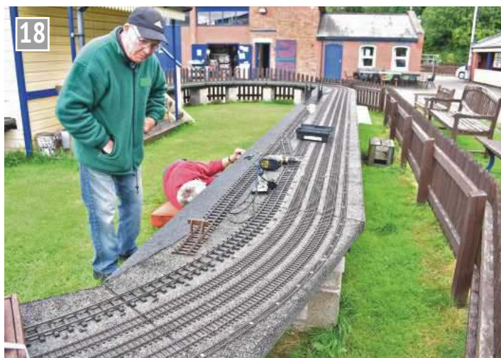
Maintenance work on the three-gauge test track.
