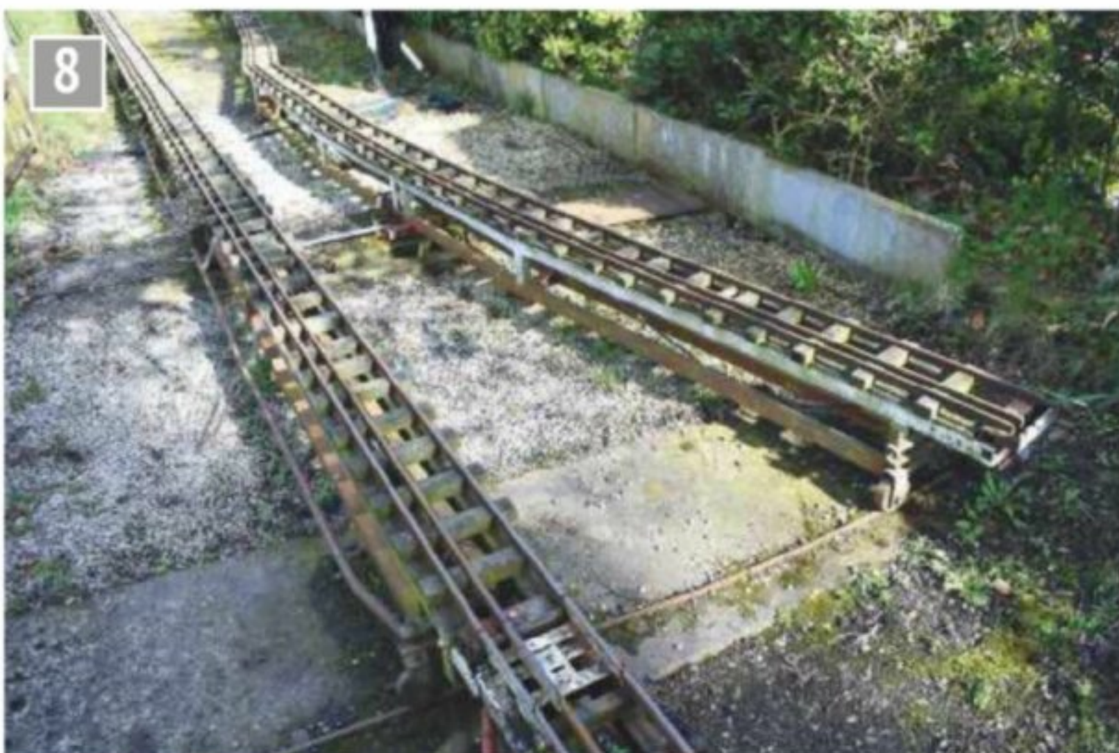
The exit traverser from the steaming bays.
