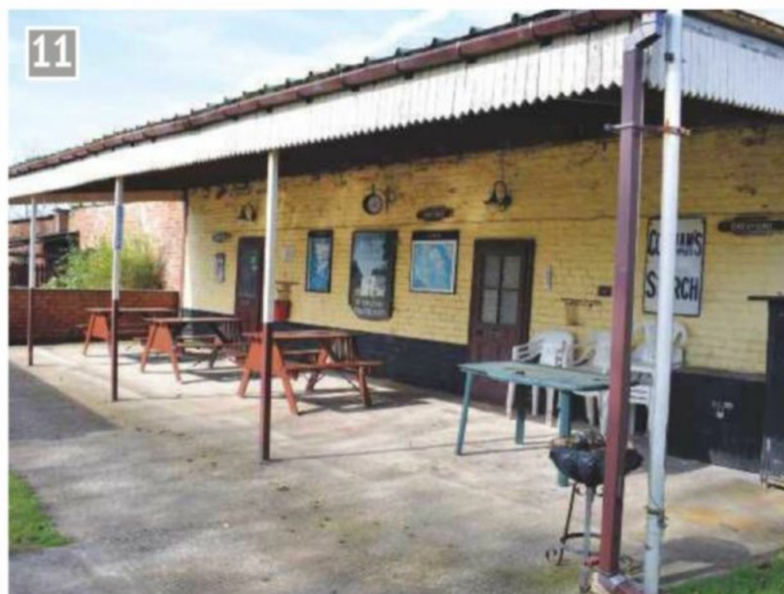
The mock station covered area.
