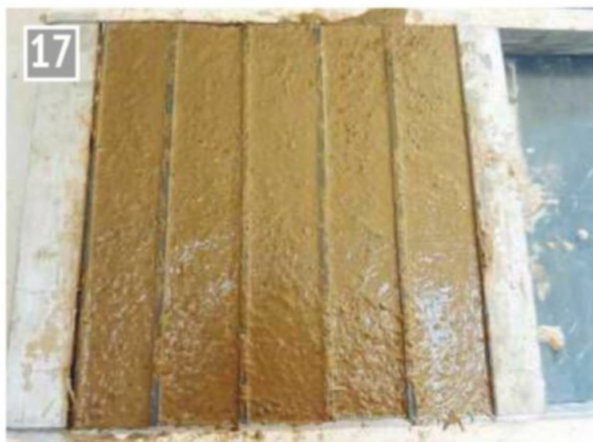
Filling is complete. Note very little bleed water at surface. This shows the water/cement ratio to be about right.
