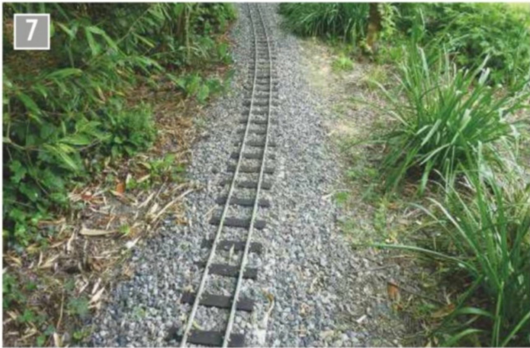
A newly laid section on concrete (just visible in foreground).
