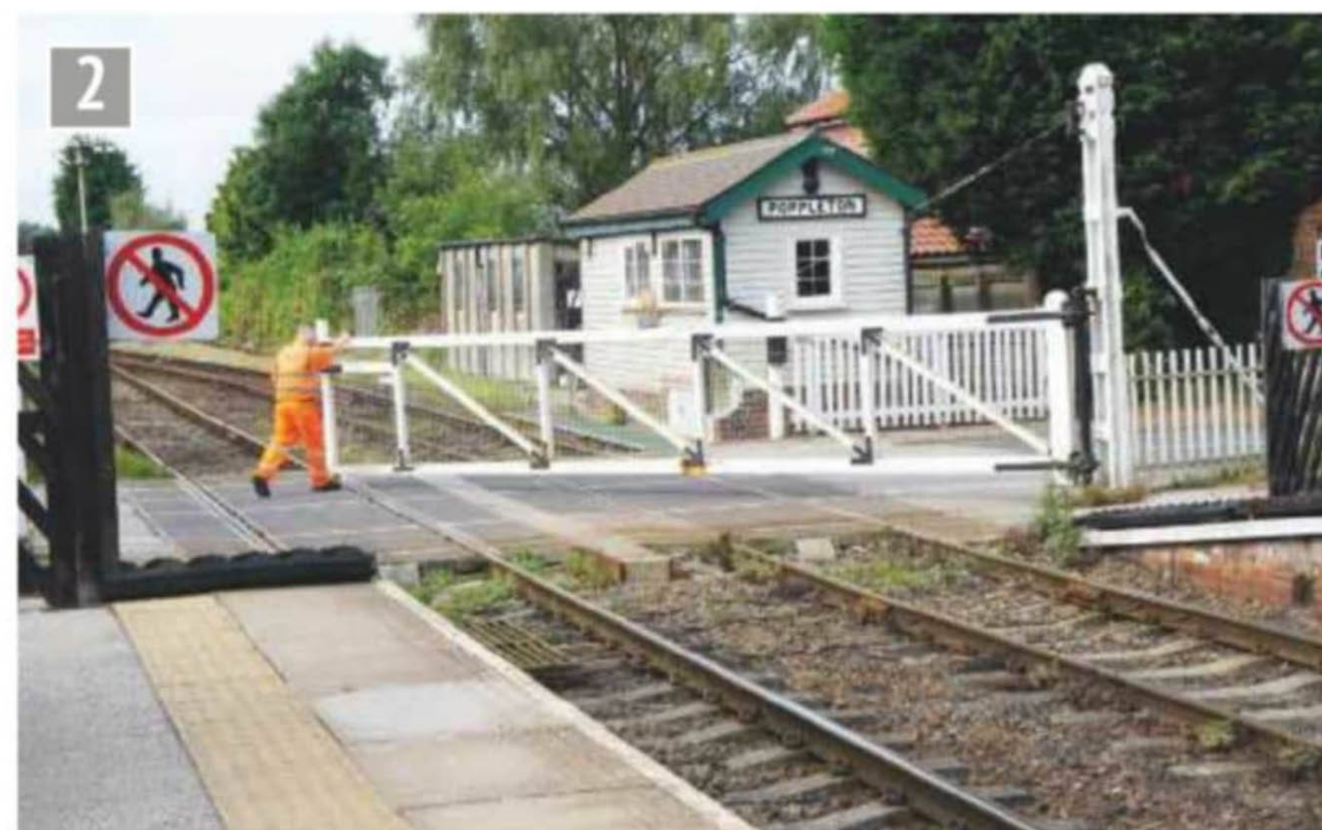
Poppleton's hand operated crossing gates and signal box. These have now been replaced by lighter metal gates.
