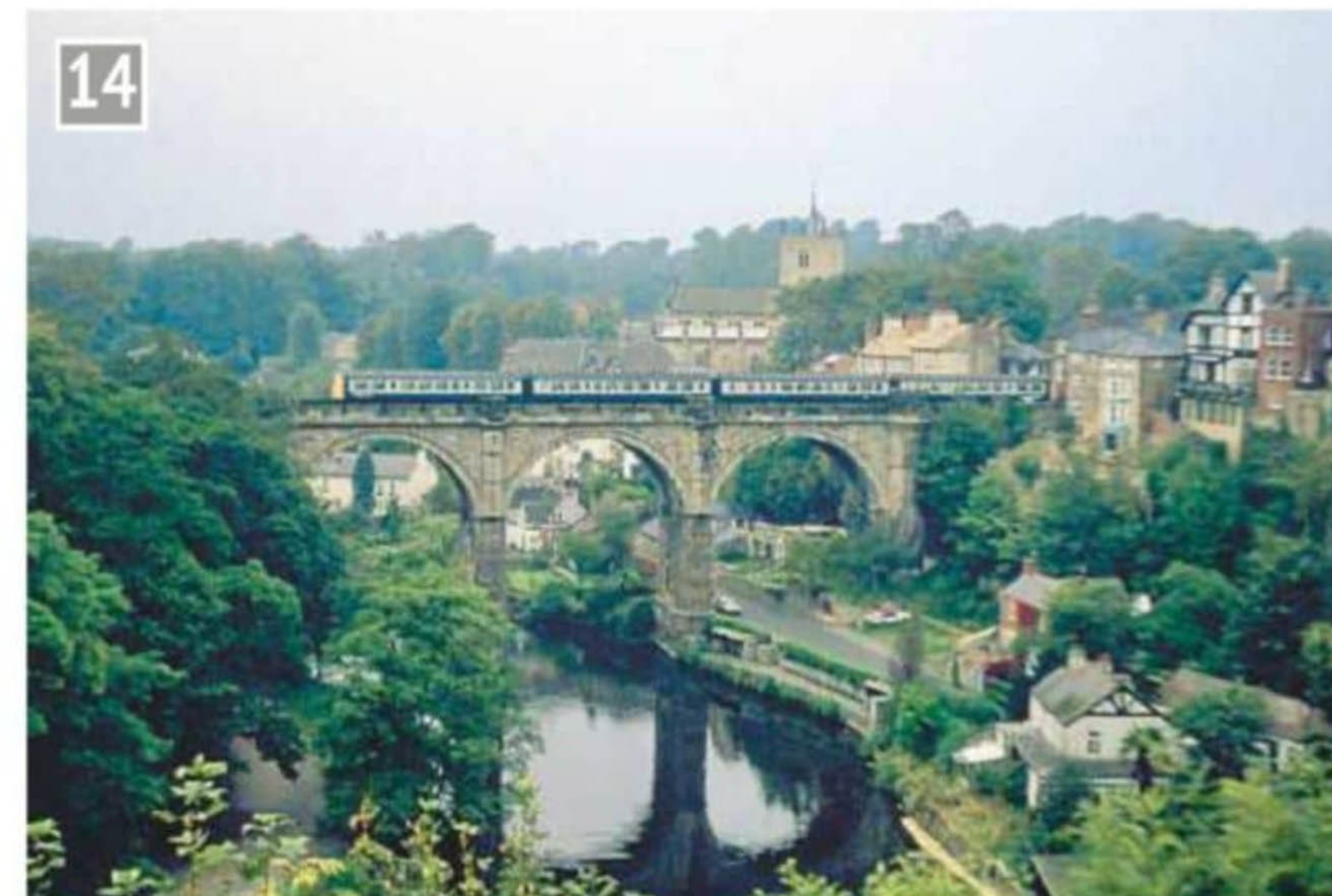
Knaresborough Viaduct seen from the castle. September 1983.
