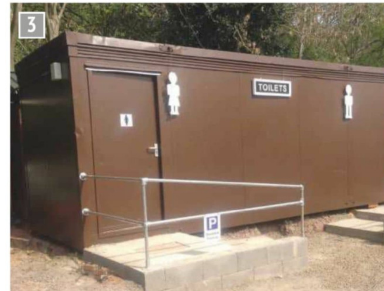
The new public toilet facilities at the Hereford SME.
