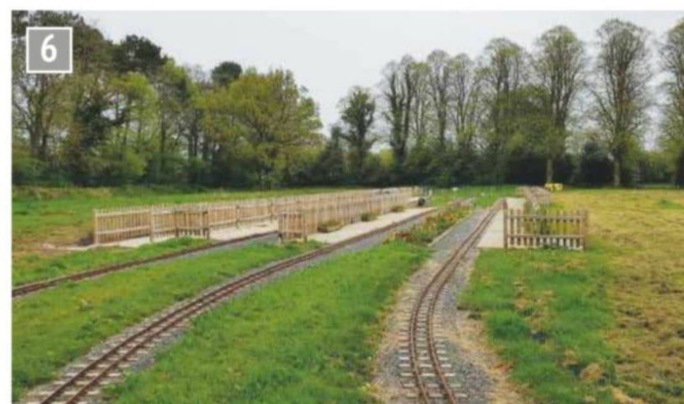
The new station at the Rugby SME under construction.
