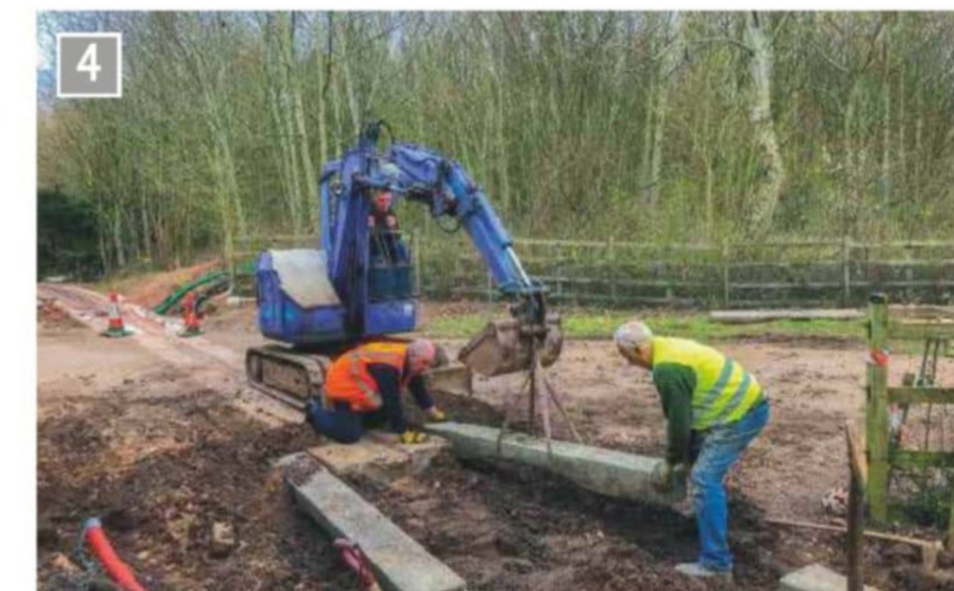
Working hard on the new extension at Nottingham.
