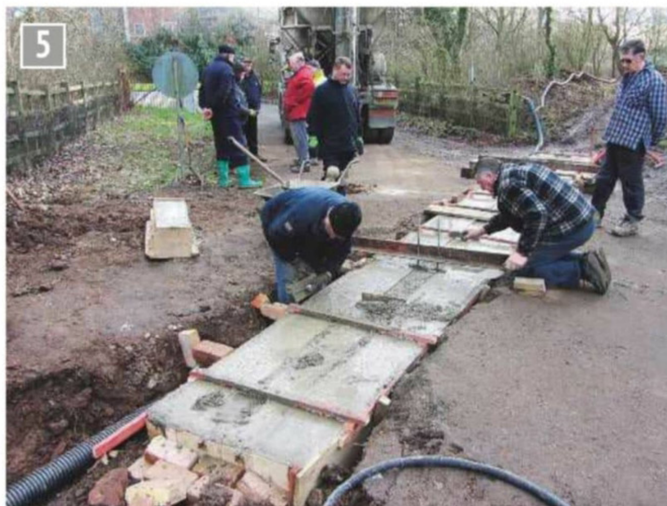
The base for the major road crossing at Ruddington is levelled out.
