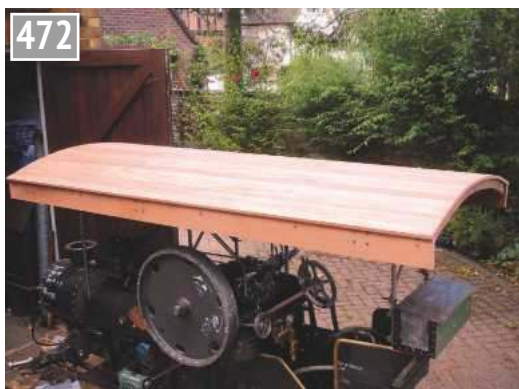
The cladding completed.
