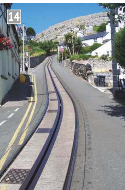
Access covers in the road surface above the rollers – always on the inside of the curves.
