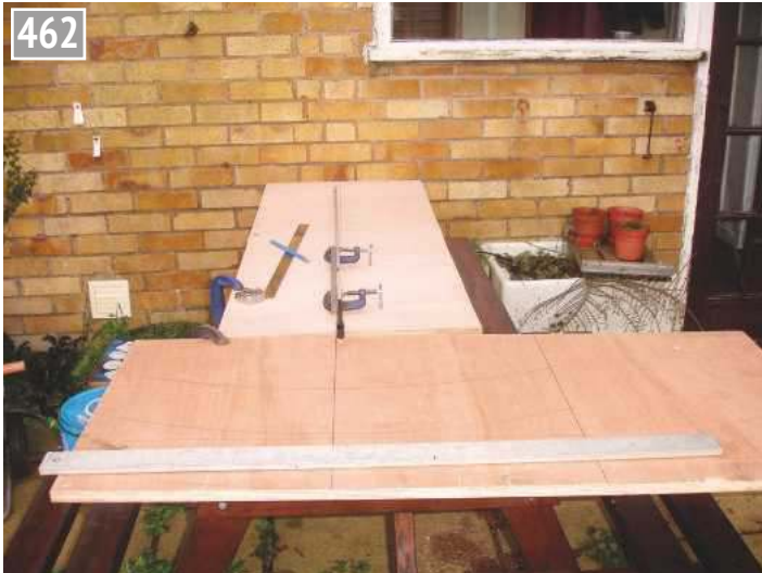
Marking out the canopy support.
