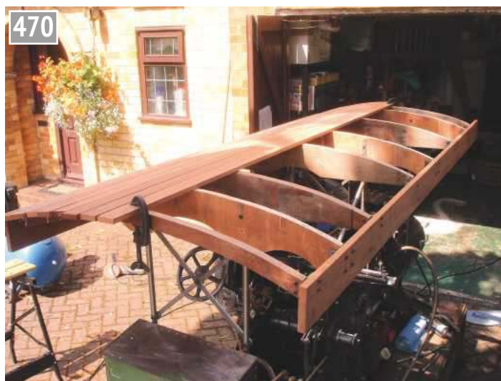
Roof cladding part complete.
