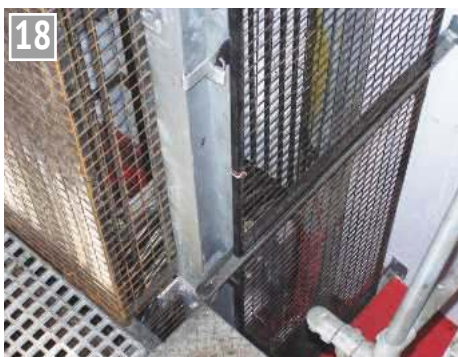
The pit is 17 feet deep!
