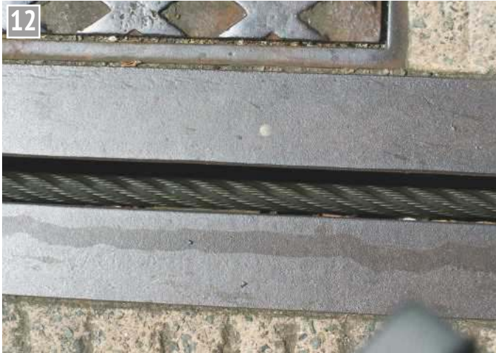
The Lower Section haulage cable.
