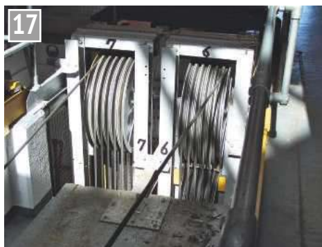
The compensating pulleys.
