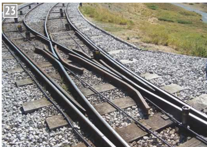
23 The check rails on the points at the top of the Upper Section passing place.
