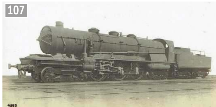
Nord Baltic with du Temple boiler, 3.1102.
