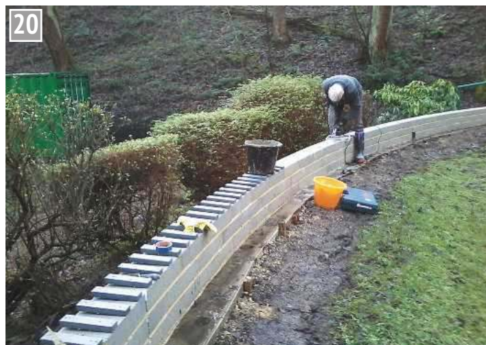
Using the jig to locate the screws for the sleepers.
