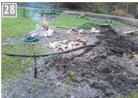
The extension to the land drain being laid into the trench.
