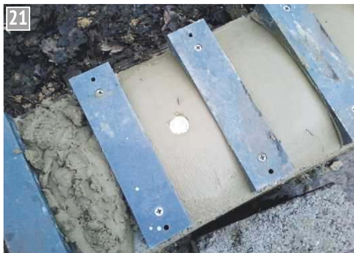
The 2017 pound coin cemented into the flaunching.
