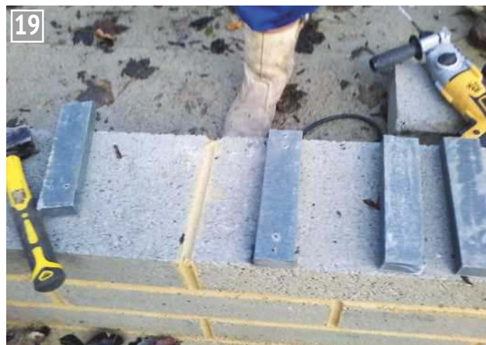
The first sleeper is screwed down.
