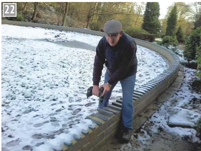
The last sleeper is fixed in position.
