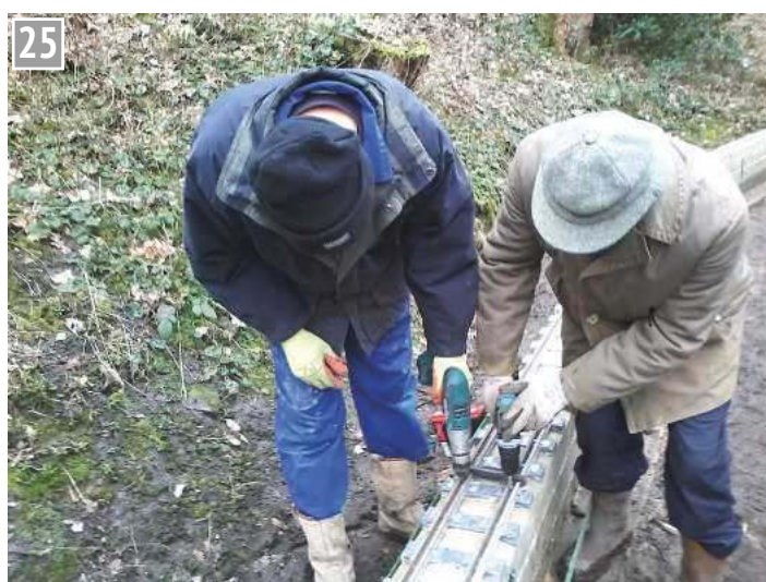
The last two screws are driven home.
