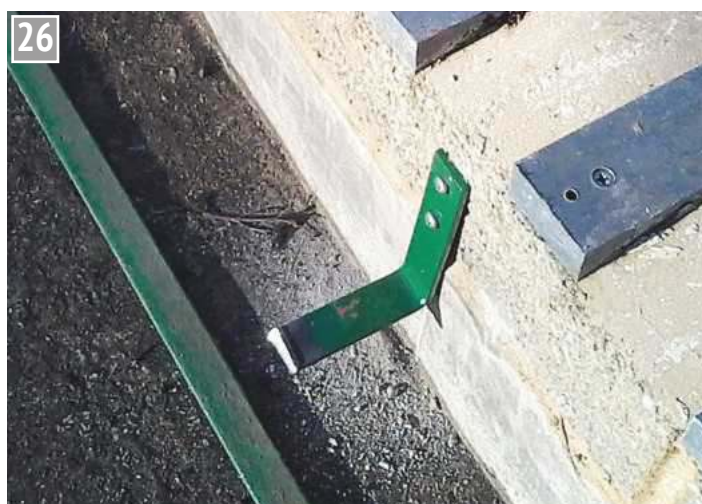
The anti-tip rail brackets fastened to the block-work.
