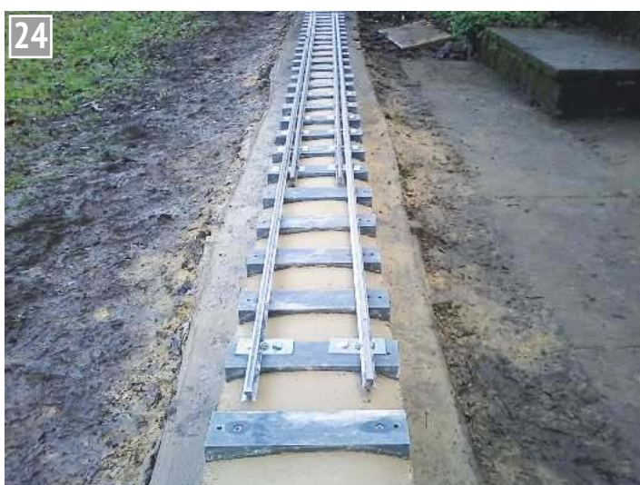
The first rails are fastened down.
