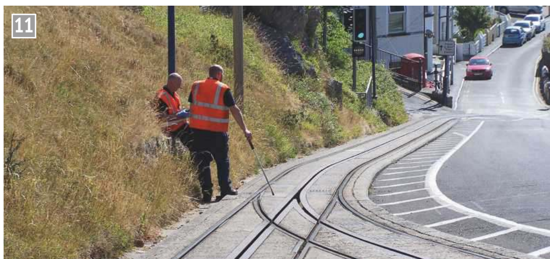
Inspecting the points to confirm they are set correctly.
