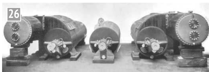
26 Turbines of SS Queen (built 1903). The high pressure turbine in the centre exhausted into the two low pressure turbines. Each of the three turbines powered a separate propeller. The cylindrical objects at the extreme right and extreme left are the condensers.
