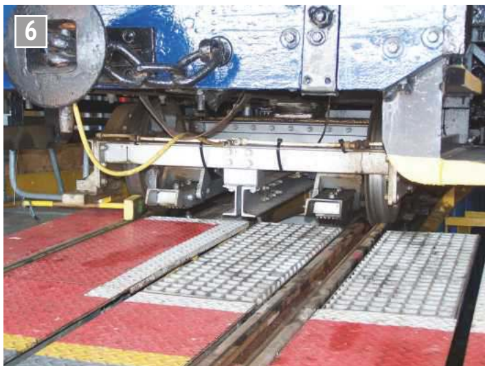
The emergency brake under the bottom of car 4.
