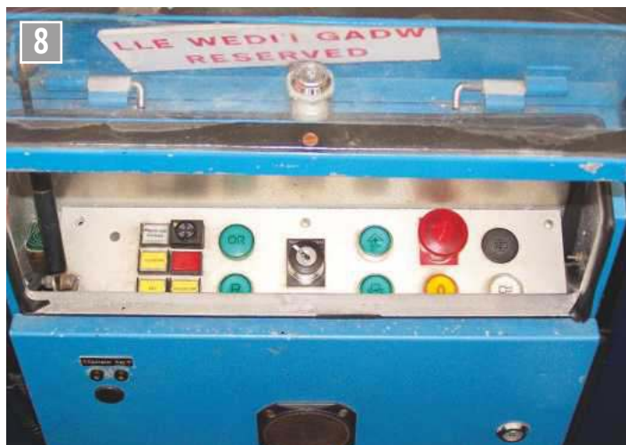
The control panel in car 4 – complete with rain cover!
