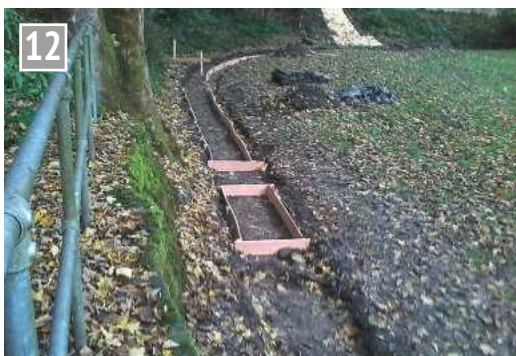
Shuttering to bridge the large tree roots.
