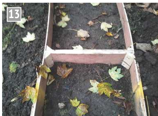
Shuttering for one of the expansion joints.
