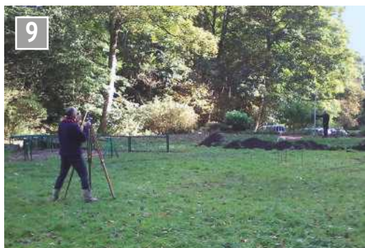
Setting out the levels for the foundations.
