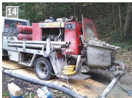
The concrete pump arrives.
