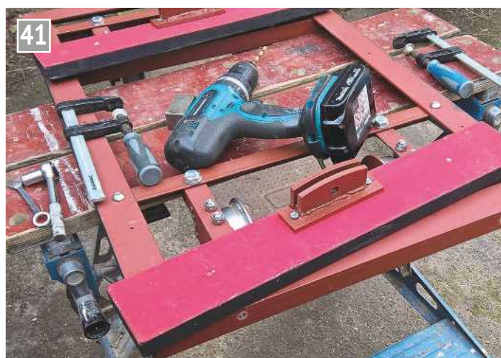
Adding the buffer beams to the frame.
