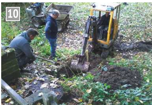
Digging out the old land drain.
