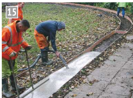
Laying and tamping the concrete up to an expansion joint.
