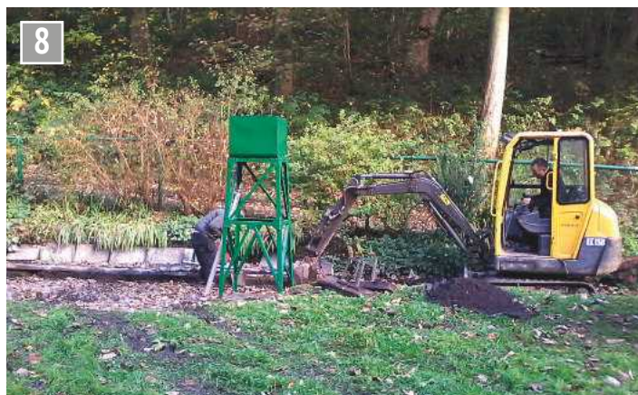
Pulling the old 'A' frames out of the ground.
