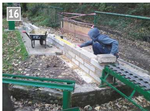
Starting the block work from the turntable.
