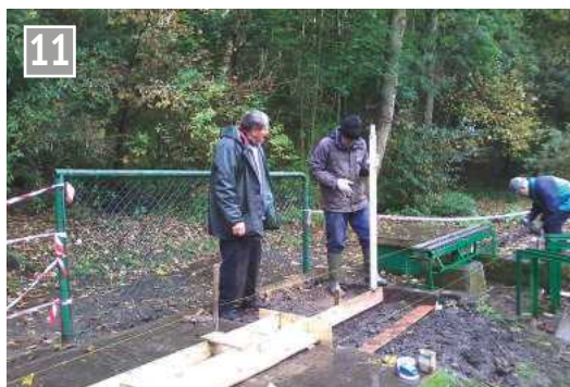
Setting the height for the shuttering to align with the turntable.
